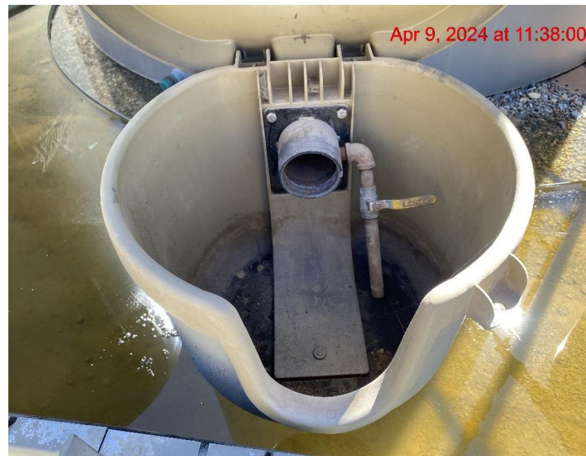
Open-Ended Load Line – Photo #00481
