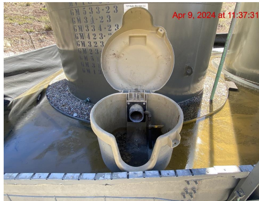
Open-Ended Load Line – Photo #00478
