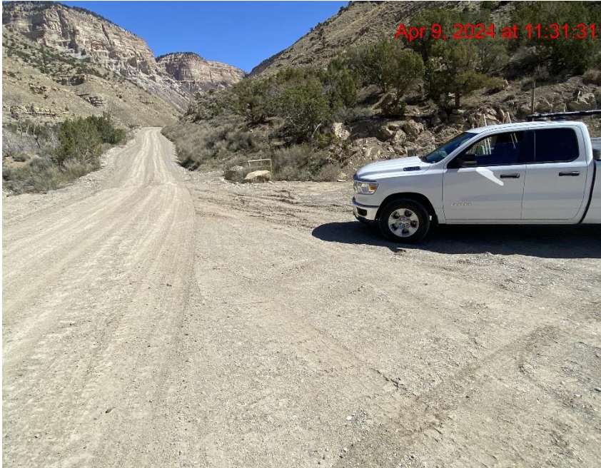
Insufficient Vehicle Tracking BMPs at Location Entrance/Exit – Photo #00470
