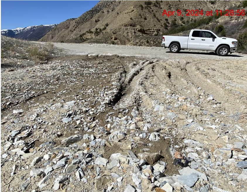
Sediment Run-on to Location/Lack of Stabilization – Photo #00465
