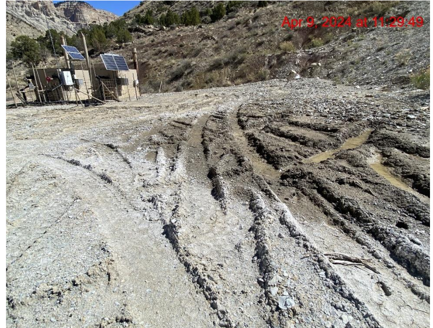
Sediment Run-on to Location/Lack of Stabilization – Photo #00467
