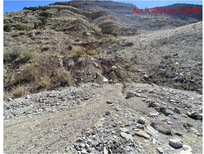
Insufficient Erosion Control/Sediment Run-on to Location – Photo #00464
