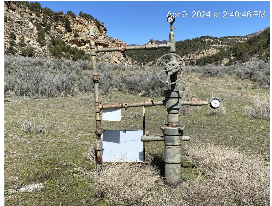
Wellhead. Stress on fittings.
