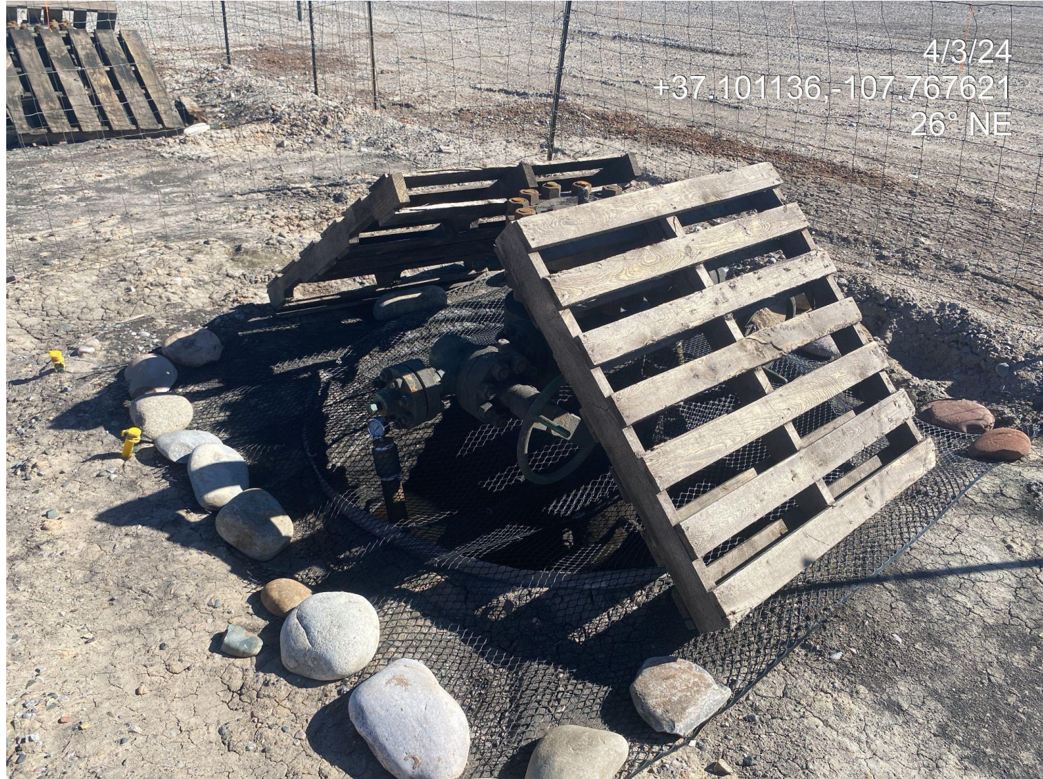
Photo 3. View of temporary wildlife BMPs/netting at the well heads.
