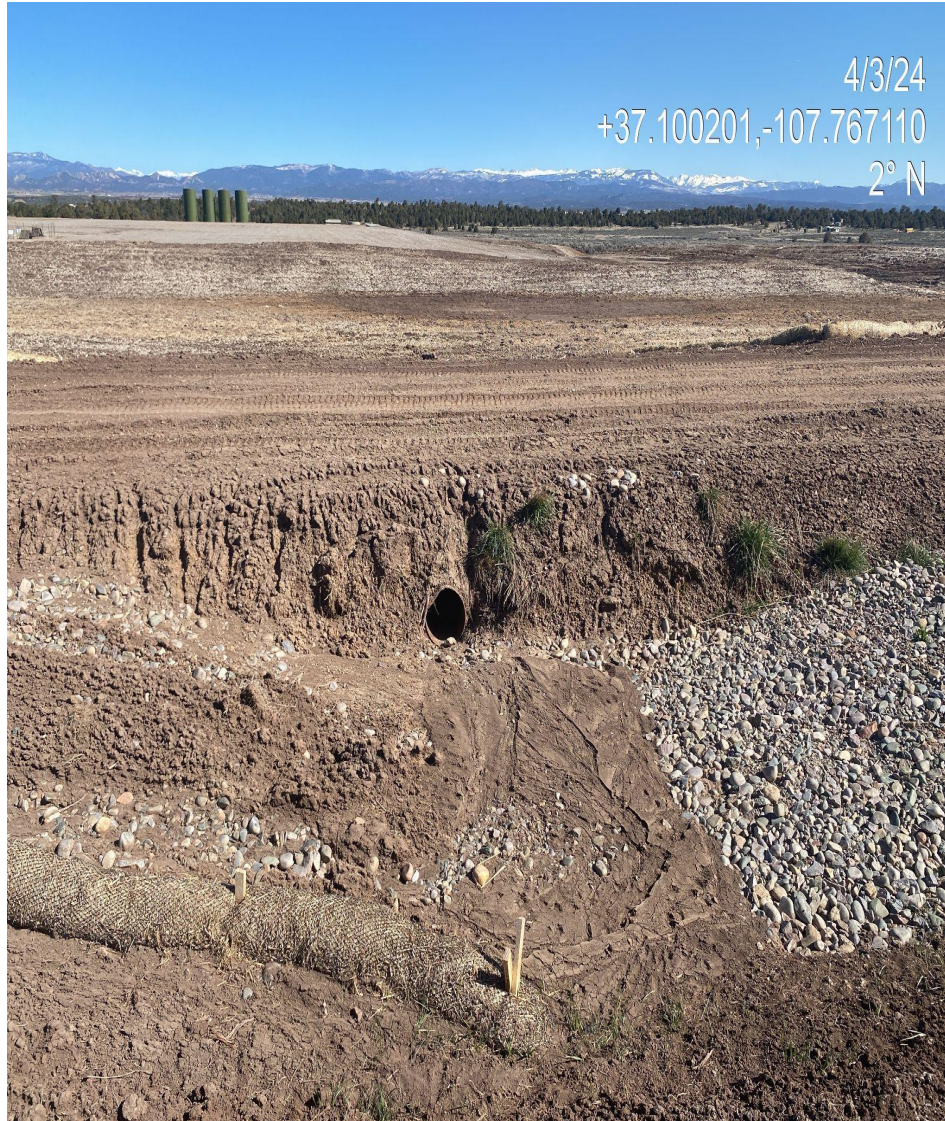
Photo 8. View of inflow and outflow of culvert built across access road that separates the southern and northern disturbances. Culvert has not been installed per good engineering practices and additional stabilization is needed.
