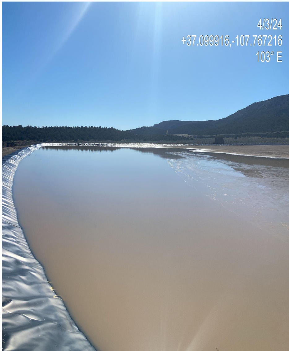
Photo 12. Storm water ponding appears evident on TUA pad. Pursuant to COA #10 a sump is planned for the northeast corner of the pad. Sump was not observed during inspection.
