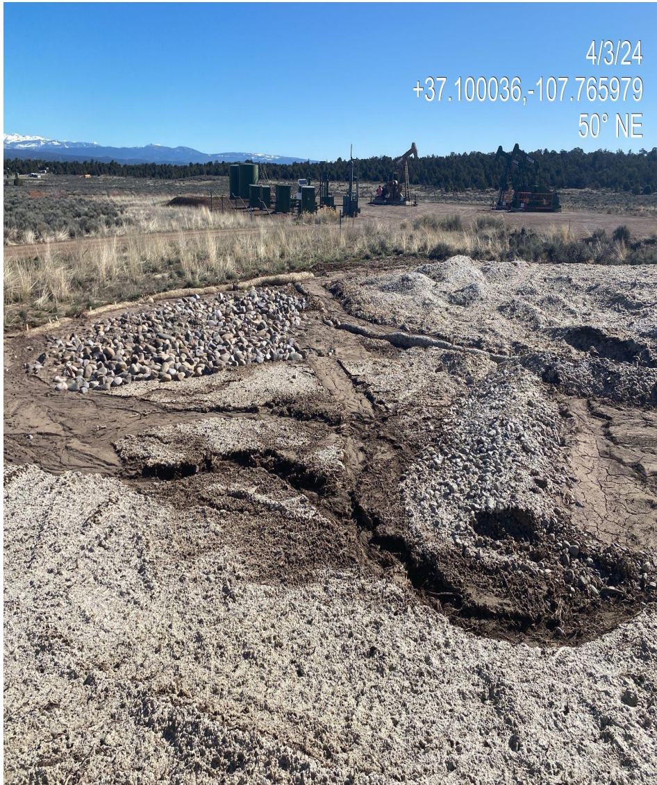
Photo 10. View of failing/inadequate stormwater BMPs in the northeast portion of the southern disturbance. Maintenance is needed in this area.
