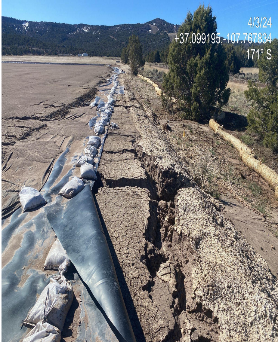
Photo 14. Gully erosion observed forming on the western edge of the southern tank pad disturbance. Maintenance is needed in this area.
