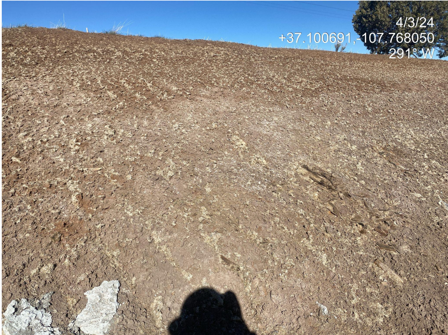
Photo 5. View of sparsely applied hydromulch/tacifier observed on the western cut slope of the well pad disturbance.
