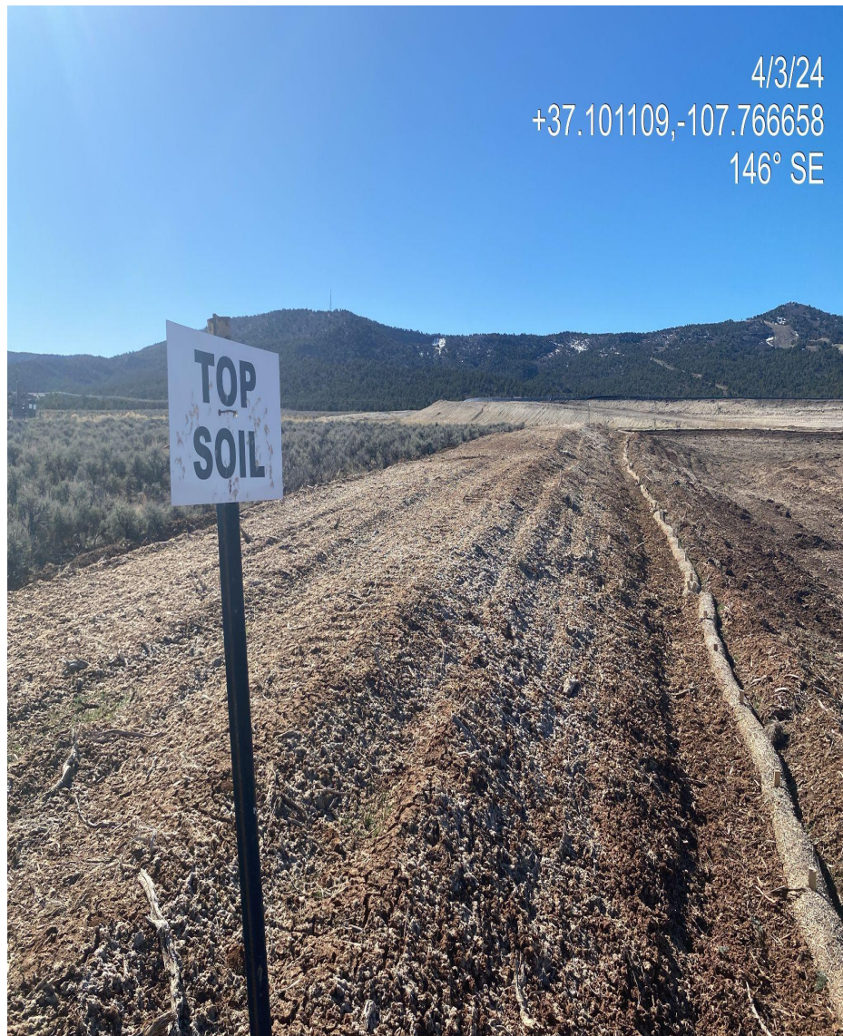
Photo 7. View of top soil stored on the eastern edge of the well pad disturbance. Sparsely applied hydro mulch/tacifier observed on the top soil salvage.
