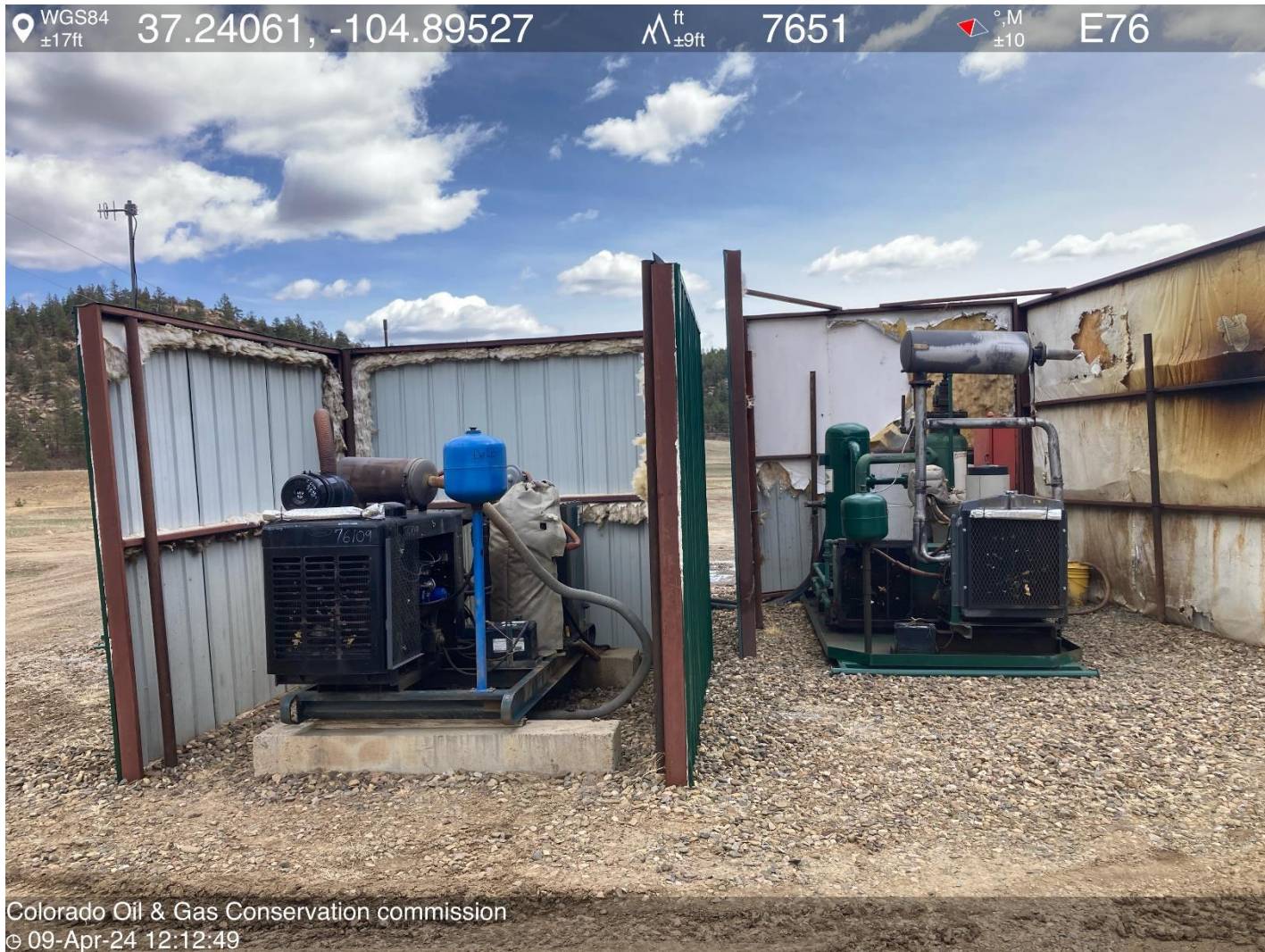
PHOTO 4: COMPRESSOR & PRIME MOVER
