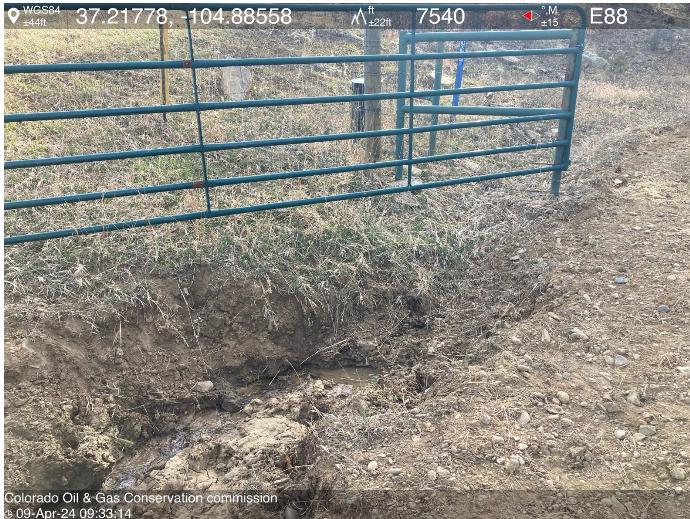
PHOTO 5: APPEARS THAT A WATER GATHERING LINE IS LEAKING APPROX. 150' NORTH OF LOCATION ALONG THE ROW. CONTACT AREA EPS CA DATE 4/11/2024.
