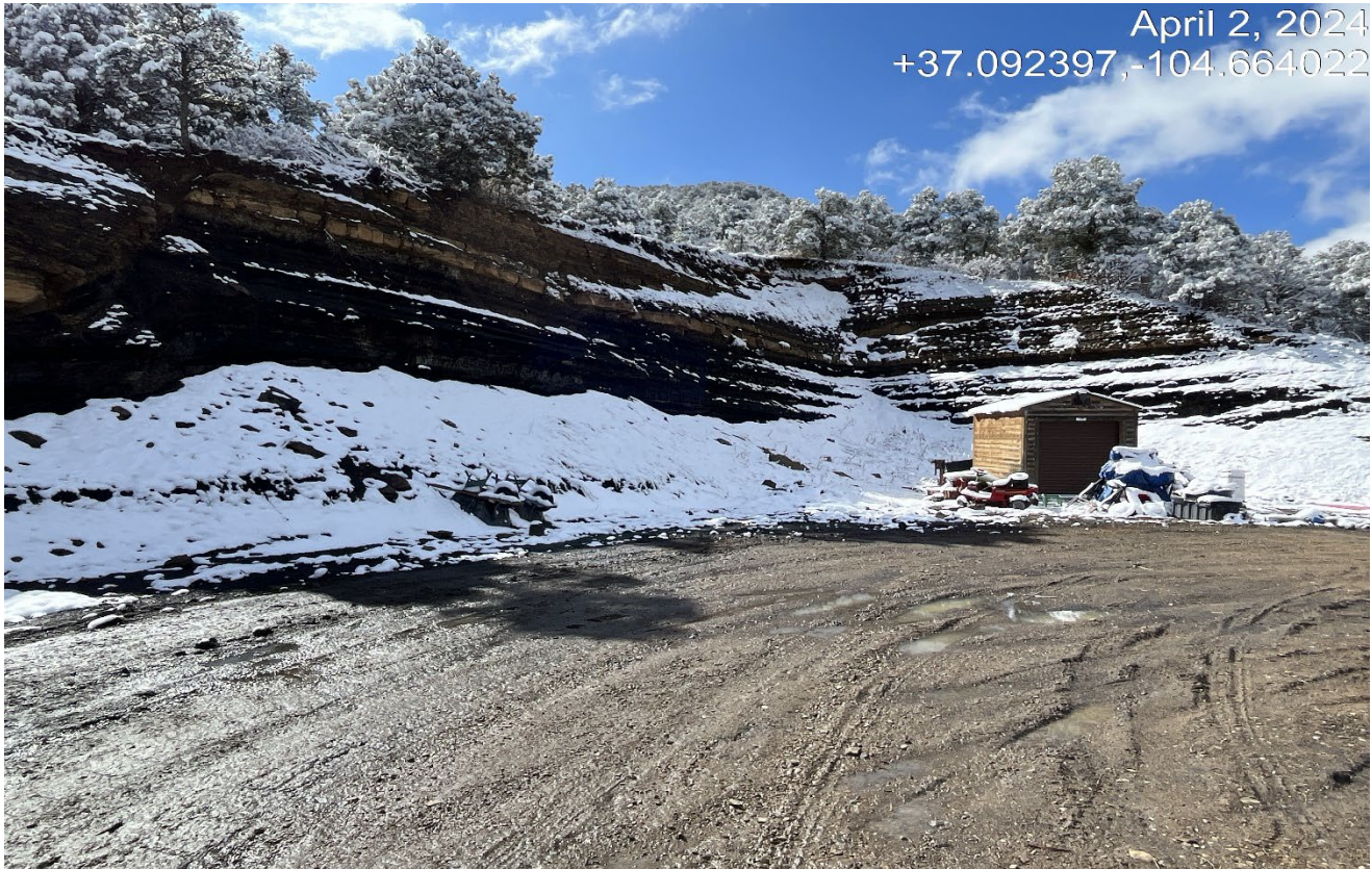
Photo 3. Facing southwest toward the vertical unstable cut slope which is approximately 50 ft. high.
