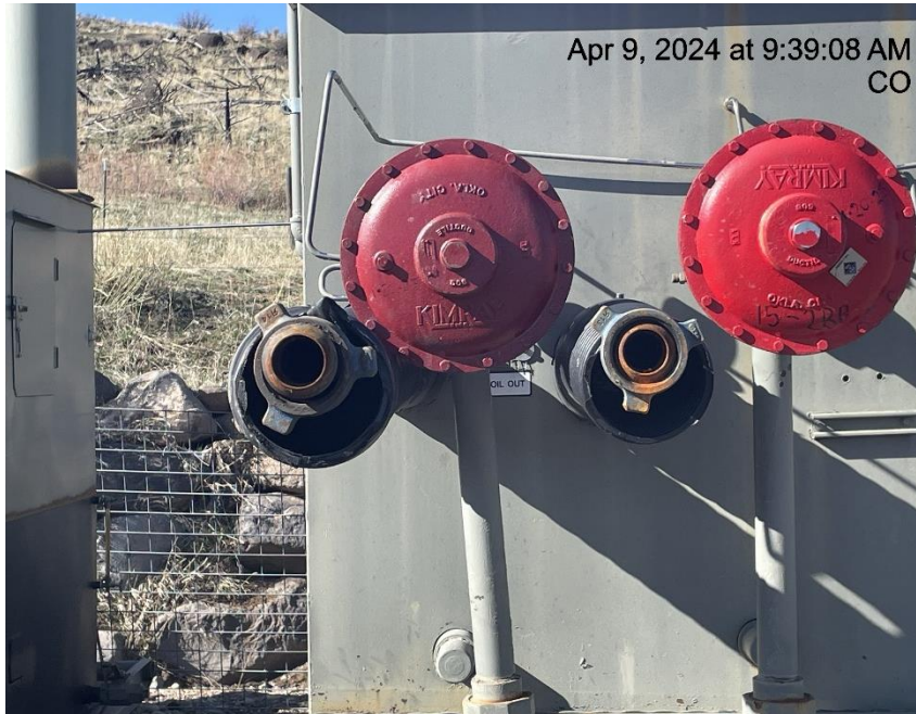
Photo # 3228 Open ended piping on separator/wildlife hazard/available for entry by wildlife
