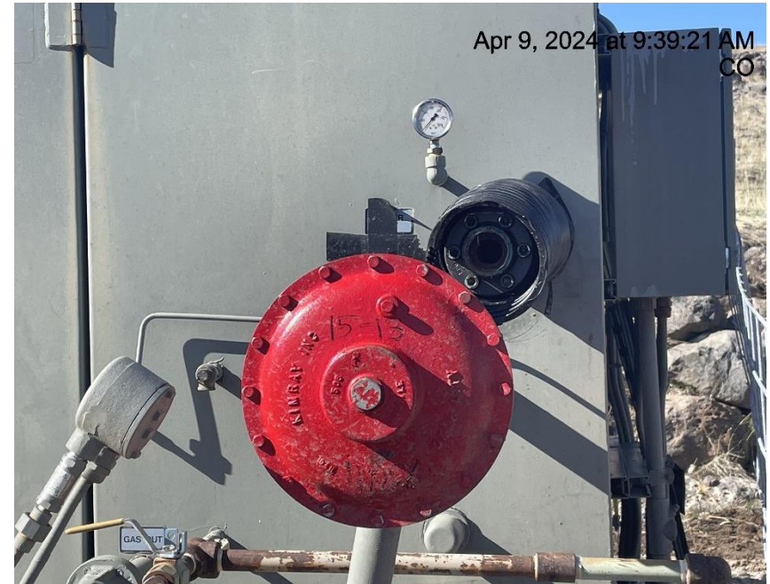
Photo # 3229 Open ended piping on separator/wildlife hazard/available for entry by wildlife
