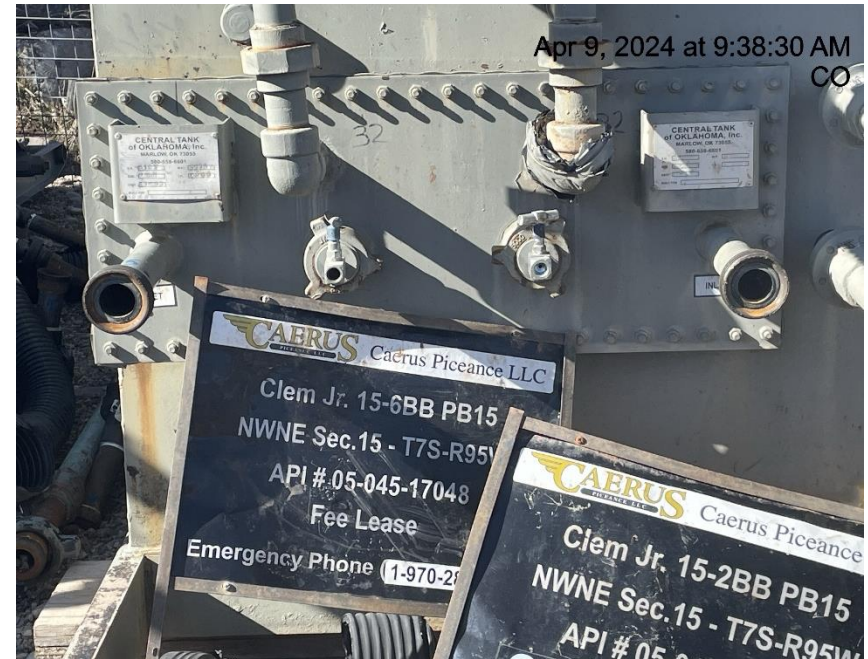
Photo # 3223 Open ended piping on separator/wildlife hazard/available for entry by wildlife
