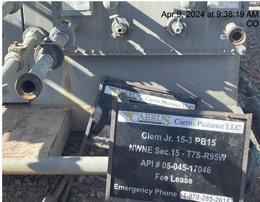
Photo # 3222 Open ended piping on separator/wildlife hazard/available for entry by wildlife
