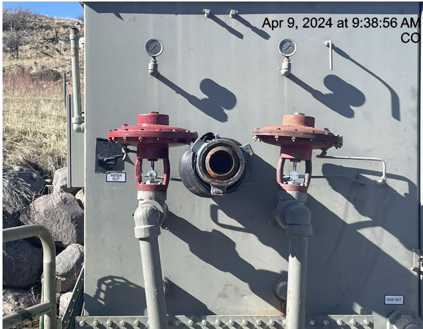
Photo # 3226 Open ended piping on separator/wildlife hazard/available for entry by wildlife
