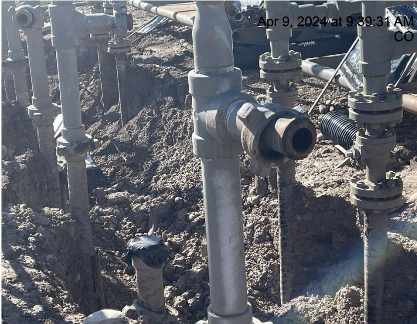
Photo # 3230 Open ended piping/wildlife hazard/available for entry by wildlife
