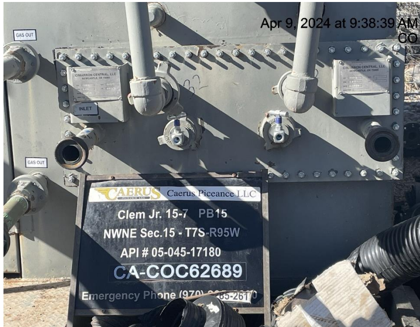
Photo # 3224 Open ended piping on separator/wildlife hazard/available for entry by wildlife
