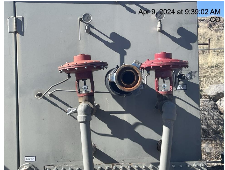
Photo # 3227 Open ended piping on separator/wildlife hazard/available for entry by wildlife
