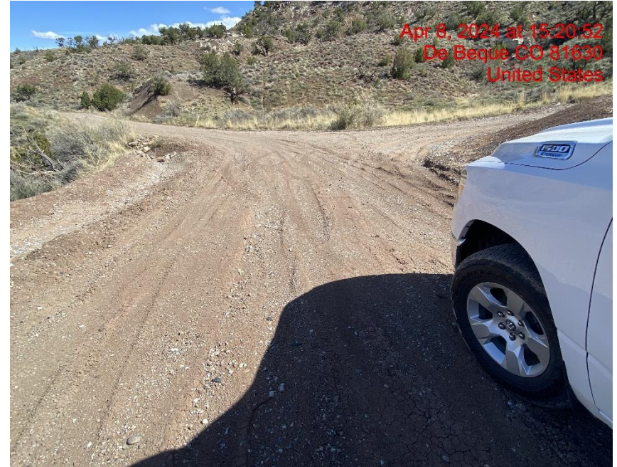
Insufficient Vehicle Tracking BMPs at Location Entrance/Exit – Photo #00451
