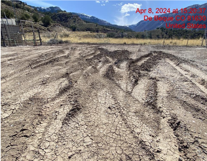
Lack of Stabilization – Photo #00450
