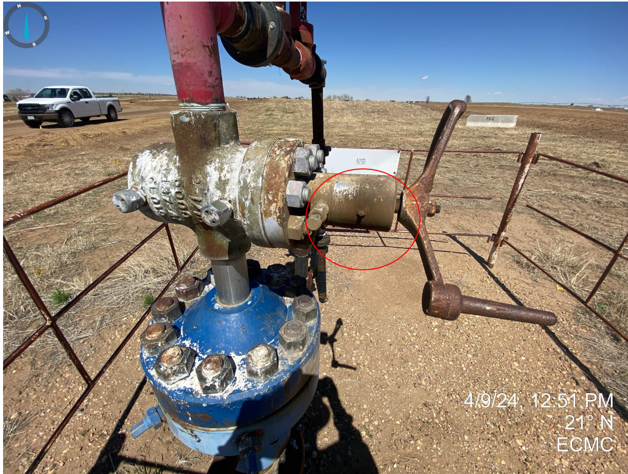
Photo 2. Approximate area where audible leak was detected.
