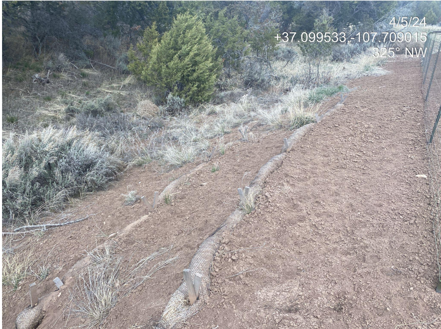
Photo 3. View of stormwater BMPs in the western portion of the disturbance that are no longer functioning. Maintenance required in this area.
