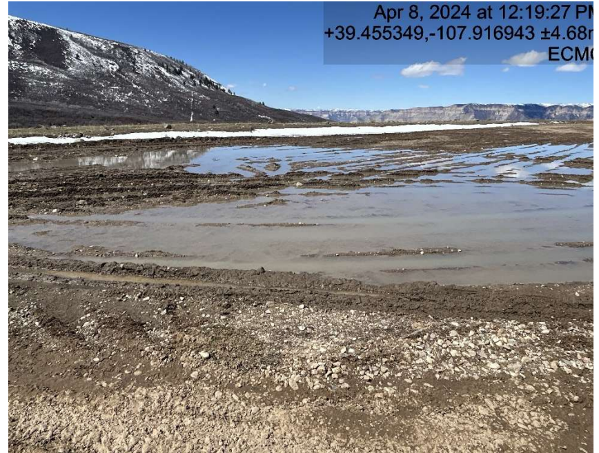
Lack of stabilization/compaction
