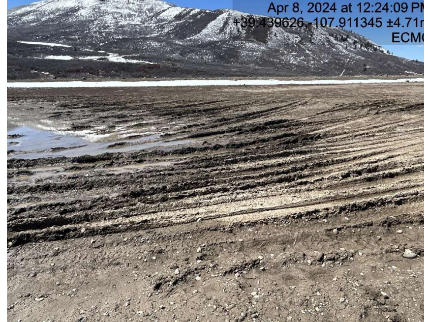
Lack of stabilization/compaction
