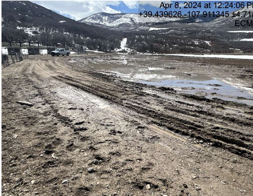
Lack of stabilization/compaction
