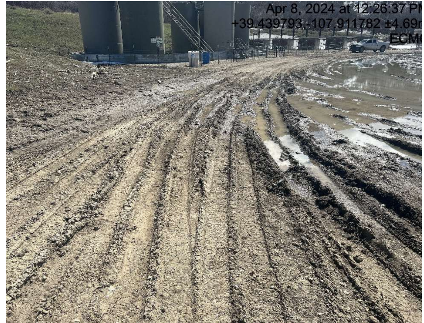
Lack of stabilization/compaction
