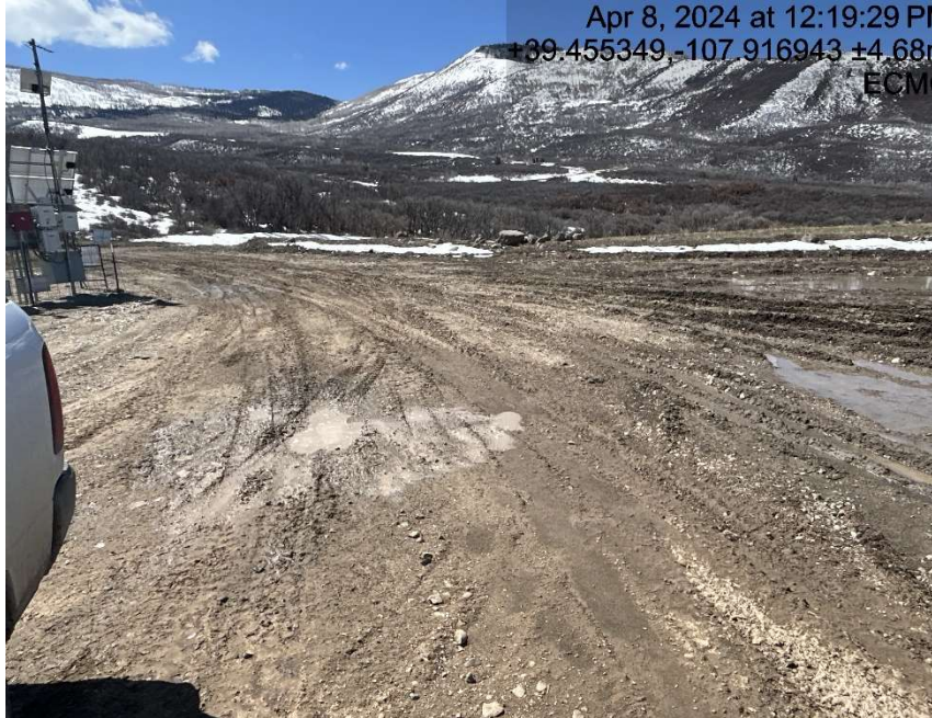
Lack of stabilization/compaction
