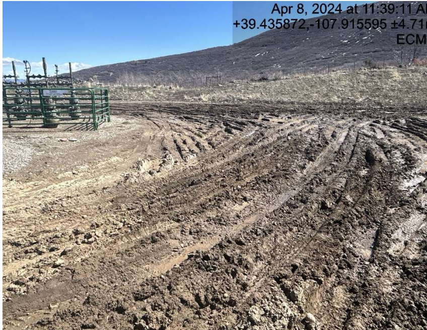
Lack of stabilization/compaction
