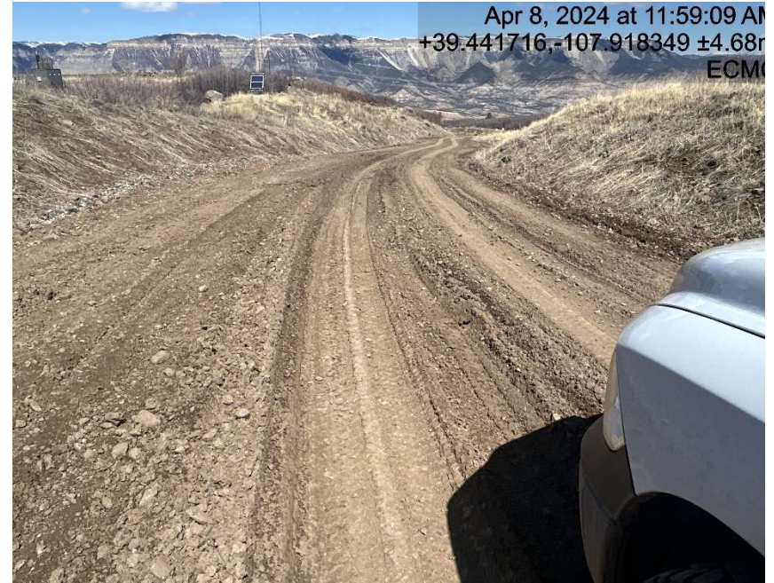
Lack of stabilization/compaction
