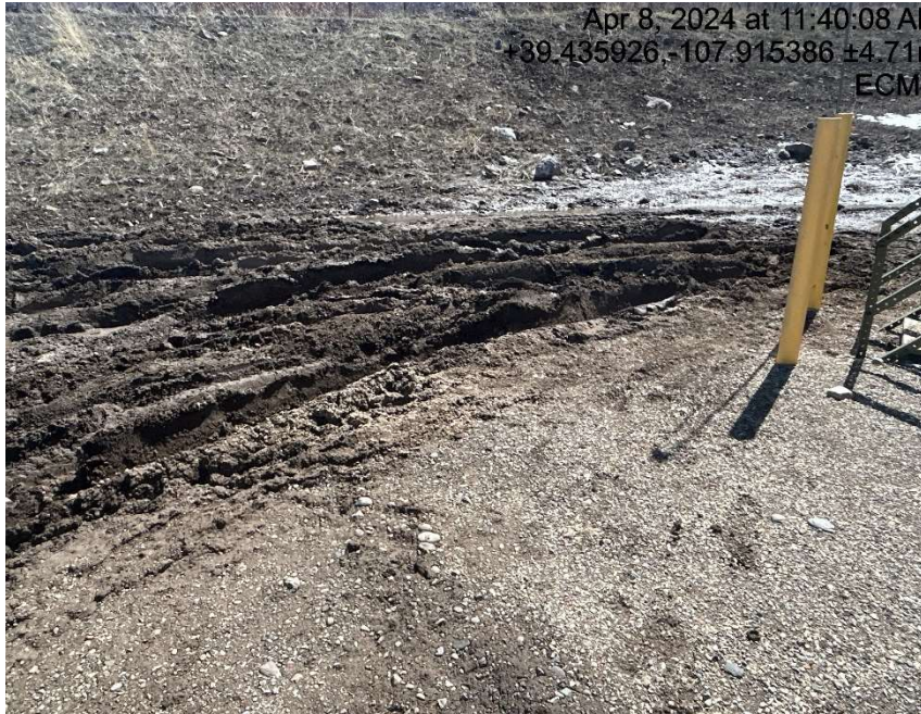
Lack of stabilization/compaction
