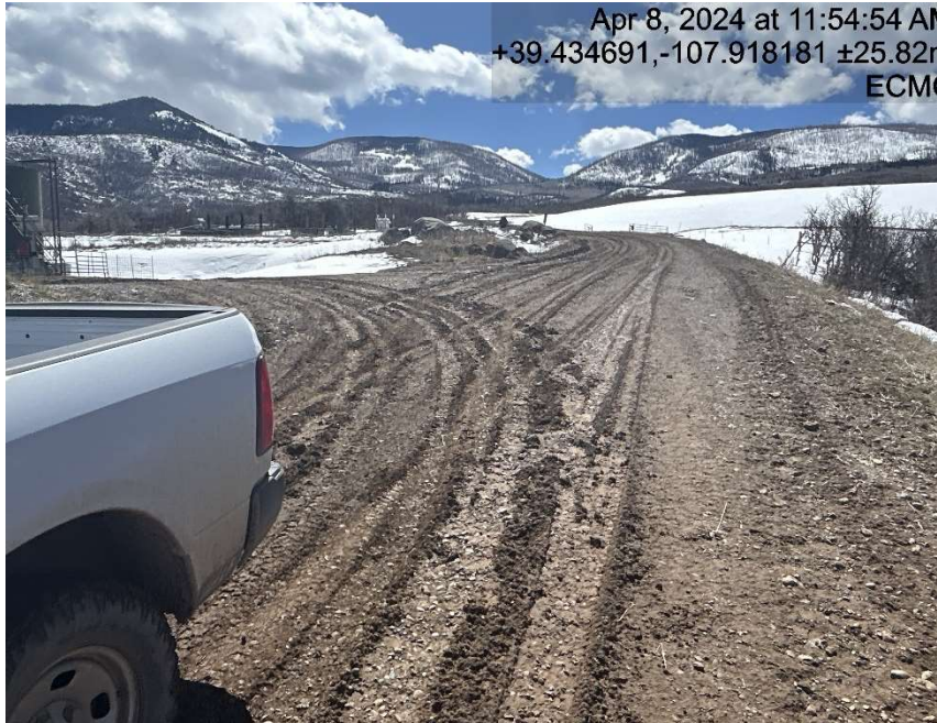
Lack of stabilization/compaction
