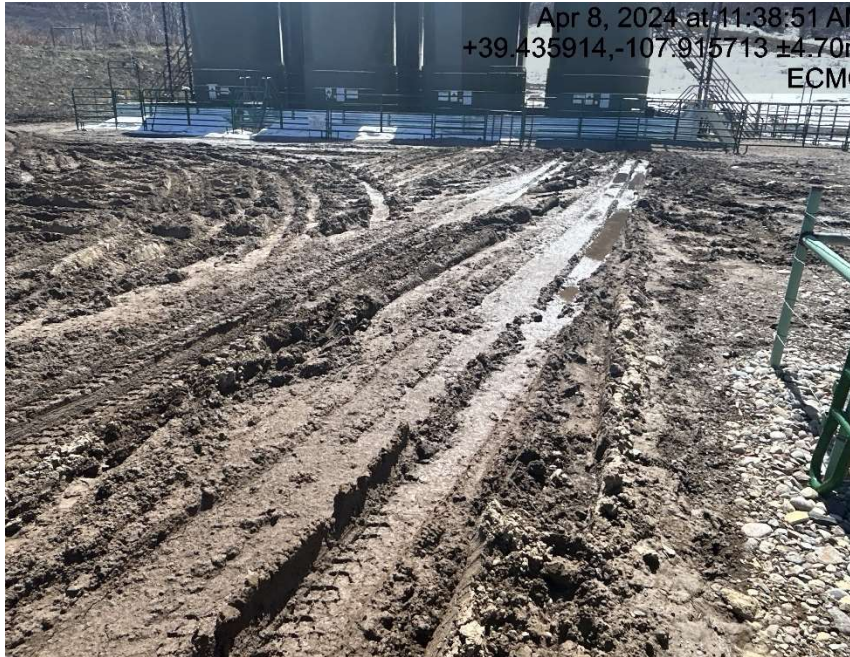
Lack of stabilization/compaction
