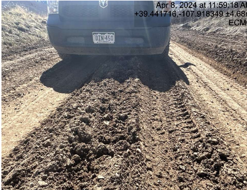
Lack of stabilization/compaction
