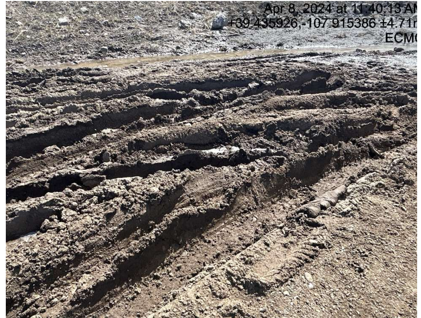
Lack of stabilization/compaction
