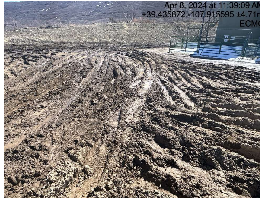
Lack of stabilization/compaction
