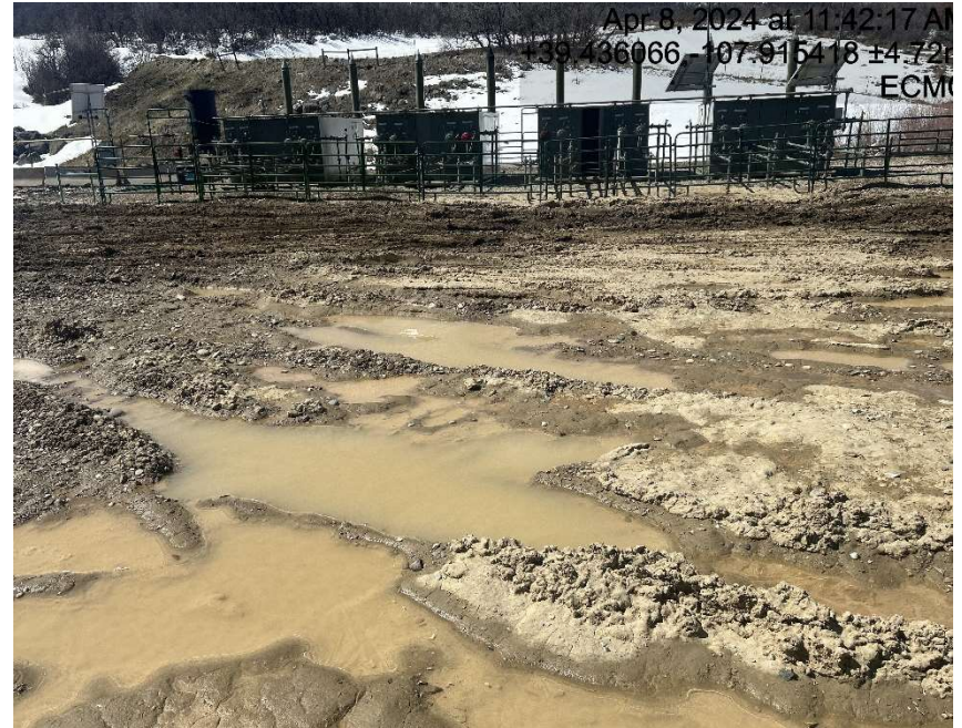
Lack of stabilization/compaction/location
