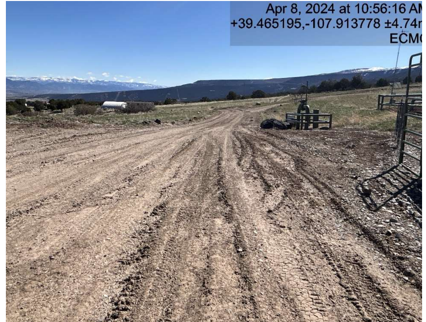
Signs of lack of stabilization/compaction
