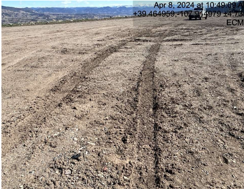
Signs of lack of stabilization/compaction
