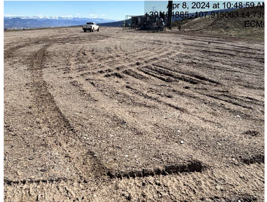
Signs of lack of stabilization/compaction
