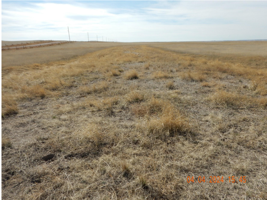
Photo 1. Photo taken from the entrance of the access road, facing West. Operator has performed final reclamation and desirable plant establishment was observed throughout the access road but there are bare patches and not uniform establishment.
