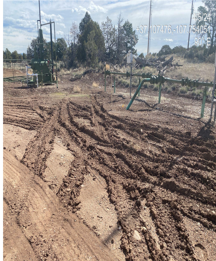
Photo 4. Rutting observed throughout the disturbance. Additional stabilization is needed to minimize site degradation. As this is shared disturbance both operators will be receiving a corrective action.
