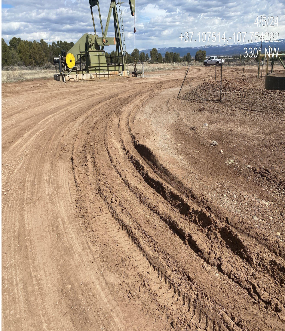
Photo 4. Rutting observed throughout the disturbance. Additional stabilization is needed to minimize site degradation. As this is shared disturbance both operators will be receiving a corrective action.
