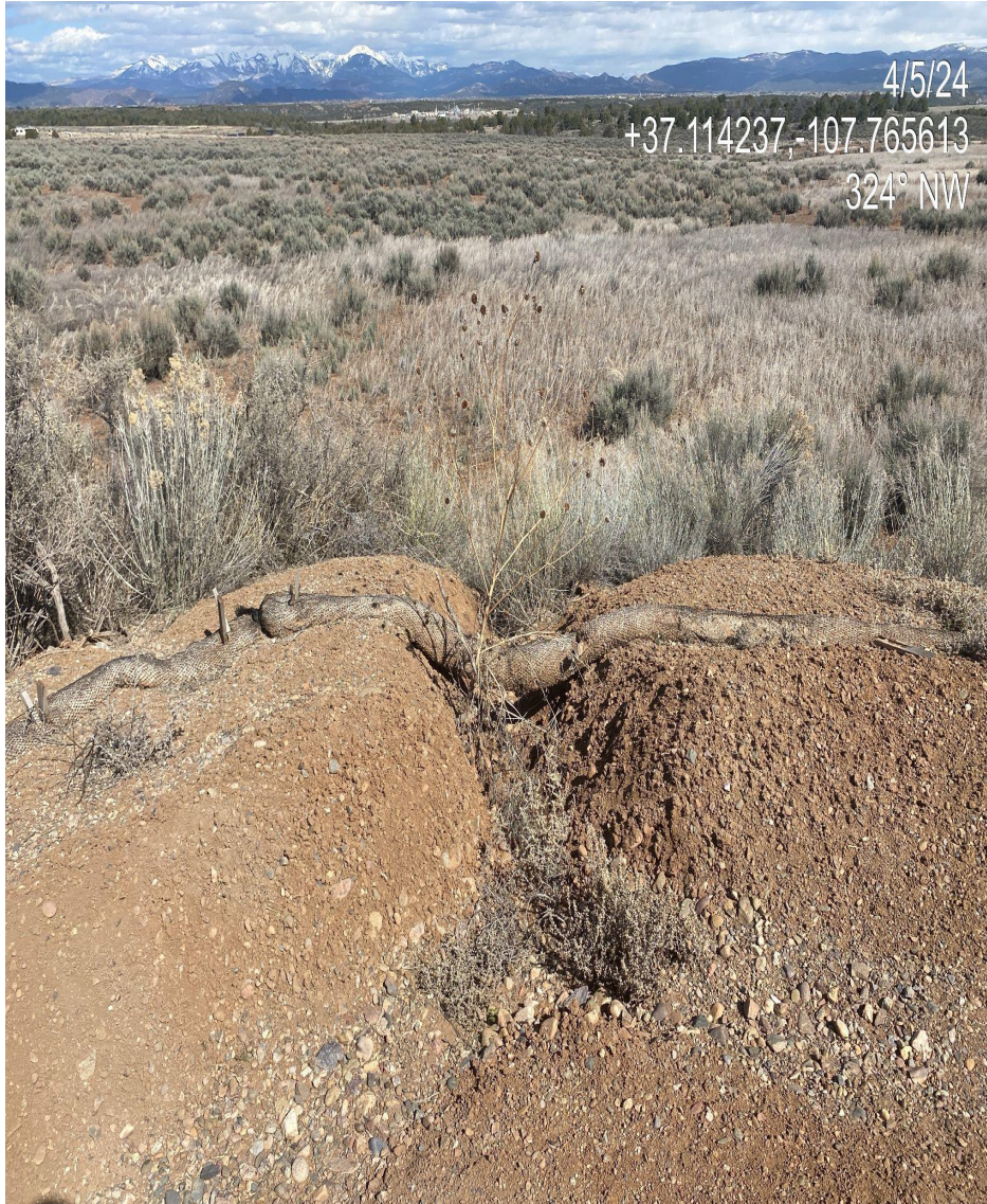
Photo 3. View of failing storm water BMPs and gully erosion forming in the northwest corner of the disturbance. Maintenance is needed in this area.
