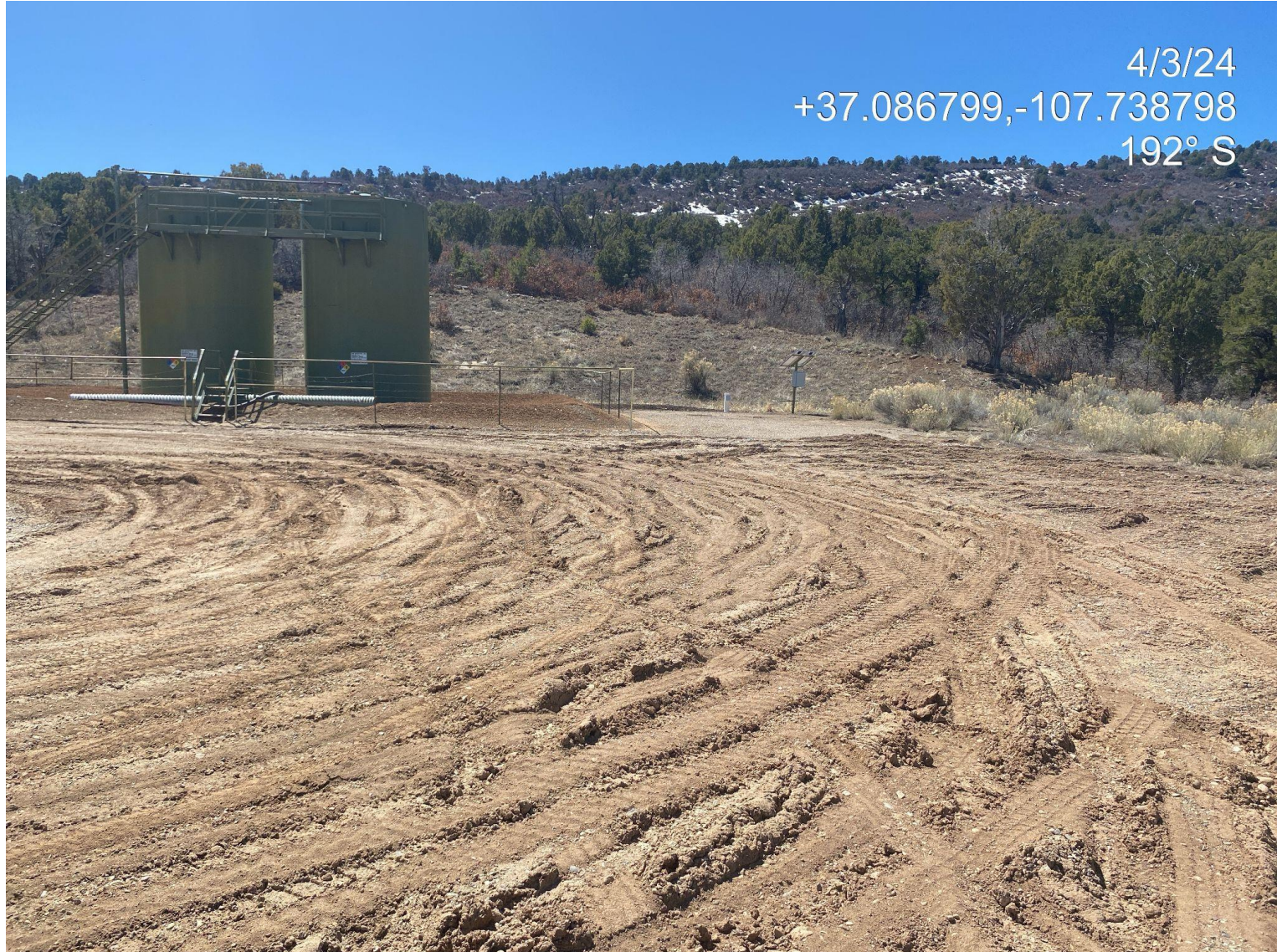
Photo 5. Rutting observed site wide. Additional stabilization is needed to minimize site degradation.
