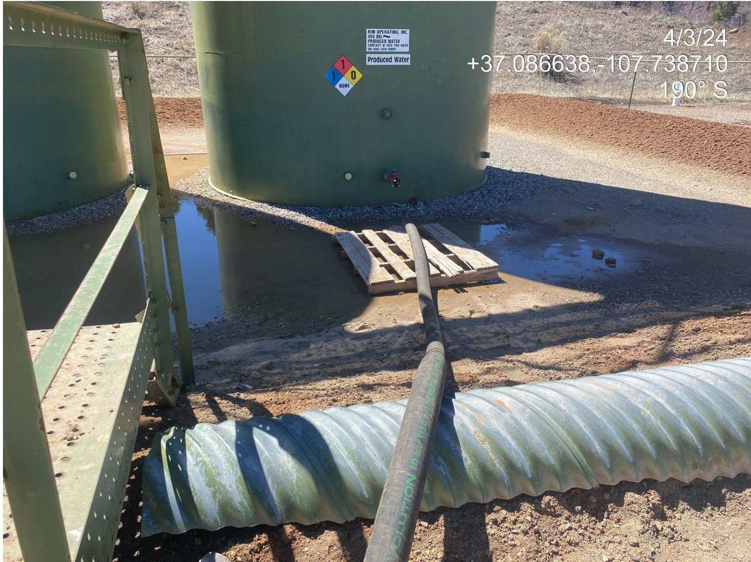
Photo 6. Unused wood pallet and culvert tubing observed stored within the produced water tanks berm.
