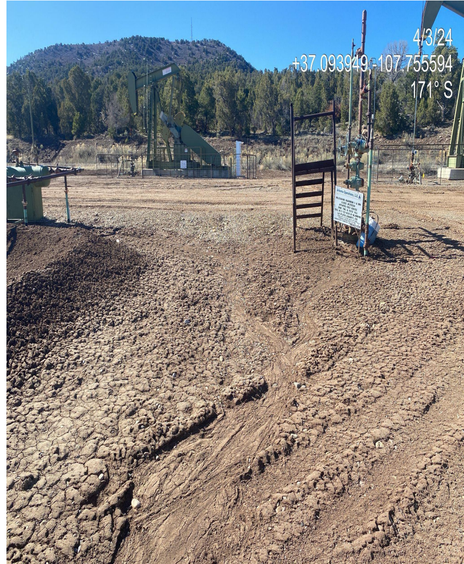
Photo 2. Evidence of sediment transport and erosion observed on location. Additional stabilization is needed.
