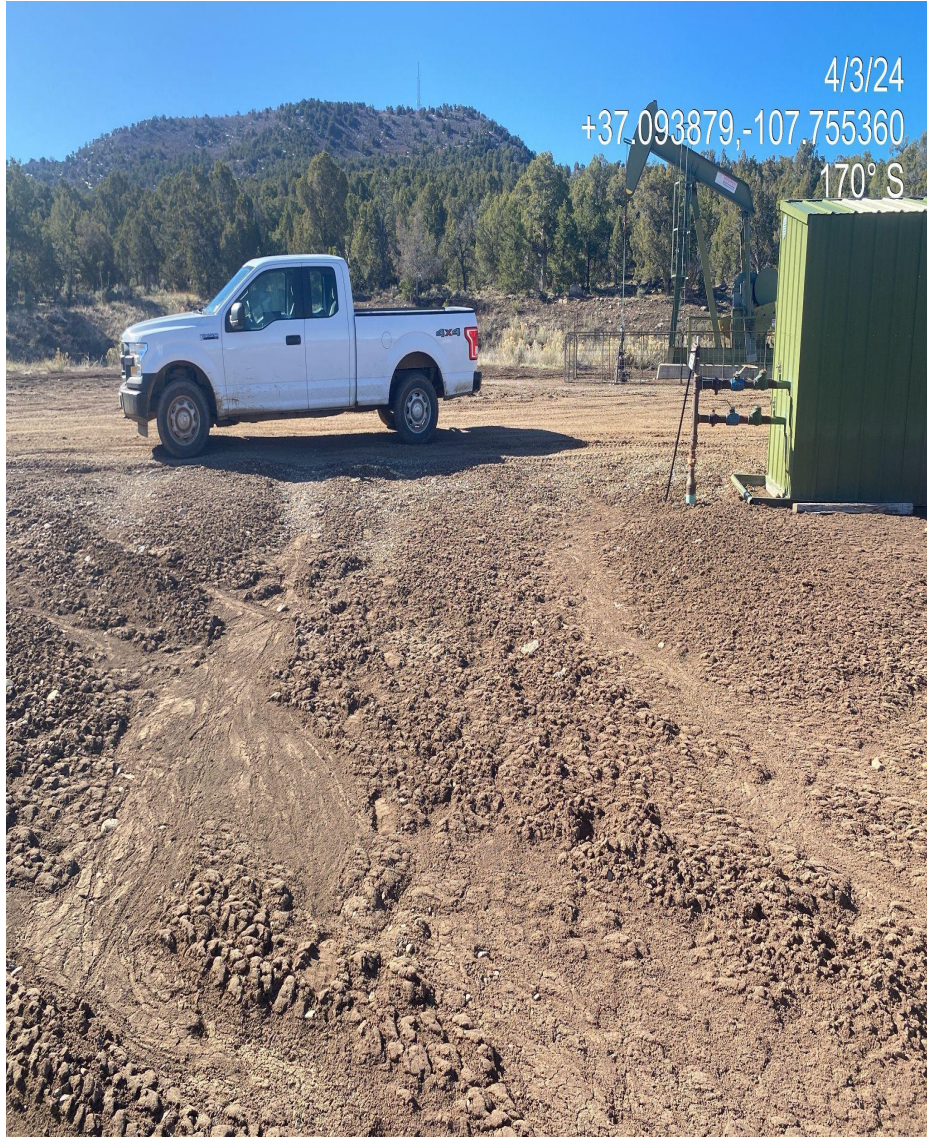
Photo 2. Evidence of sediment transport and erosion observed on location. Additional stabilization is needed.
