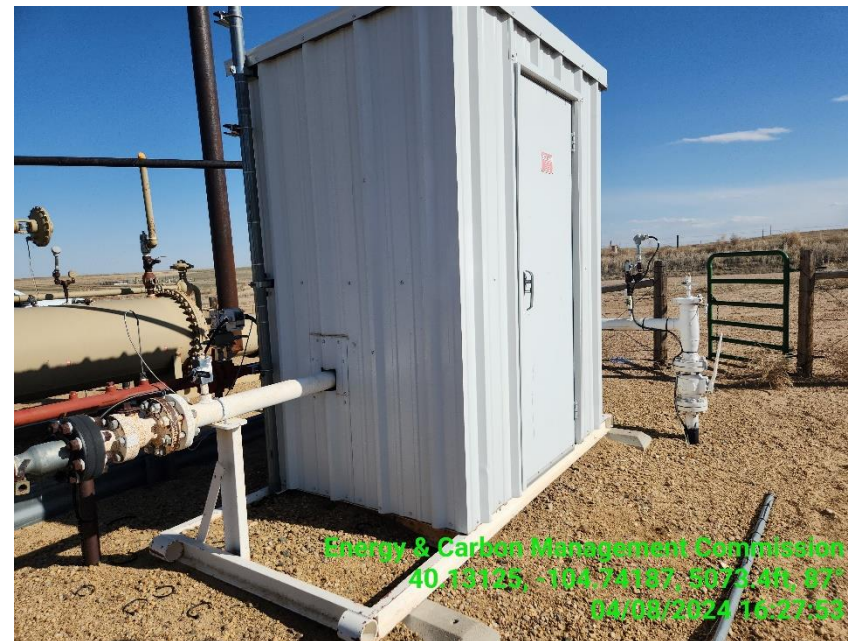
Photo 6 Gas Meter Run.
