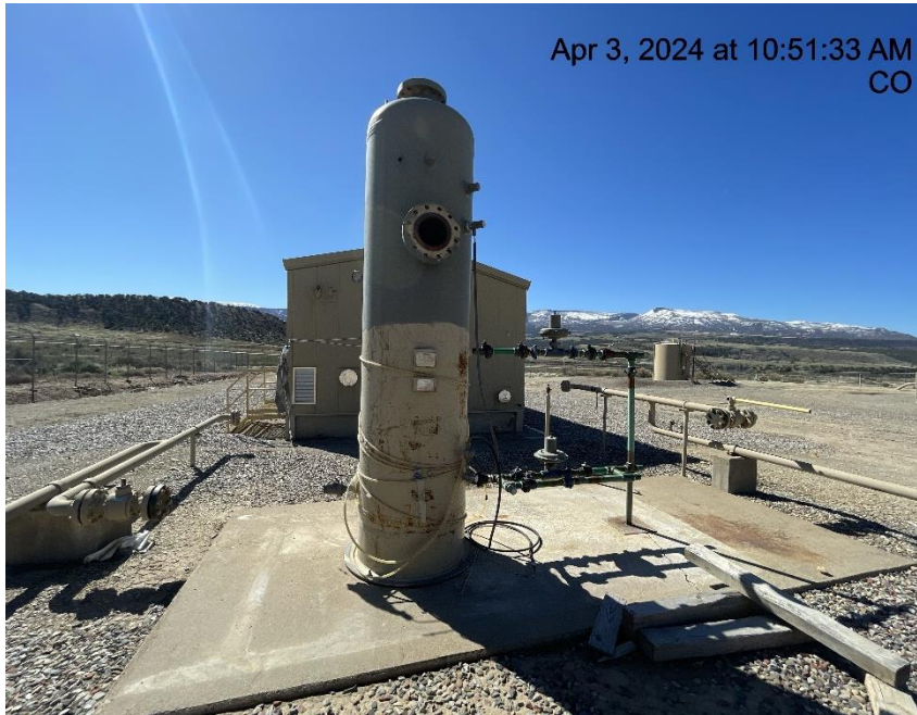
Photo # 2458 Openings on vessel available for entry by wildlife/wildlife hazards
