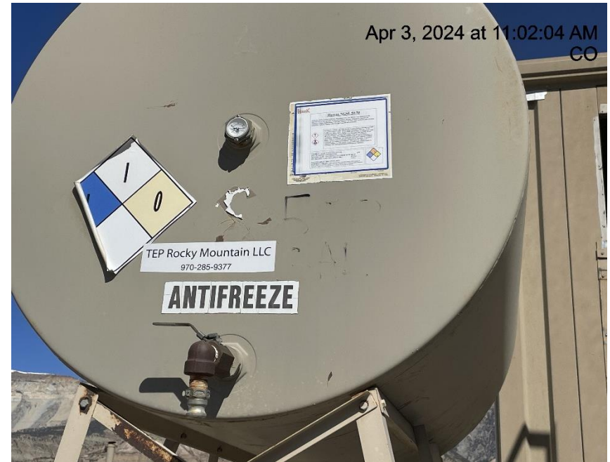
Photo # 2457 Some required info on antifreeze tank is illegible
