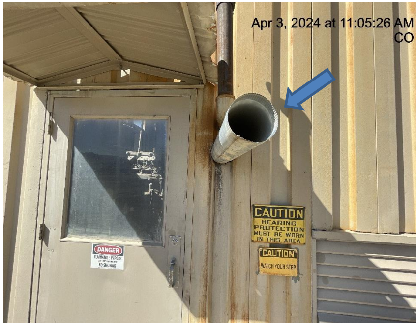
Photo # 2456 Compressor line lacks wildlife protection /wildlife hazard/available for entry by wildlife
