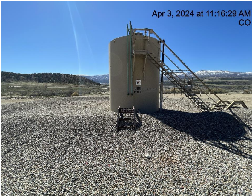
Photo # 2454 Tank battery lacks required signage
