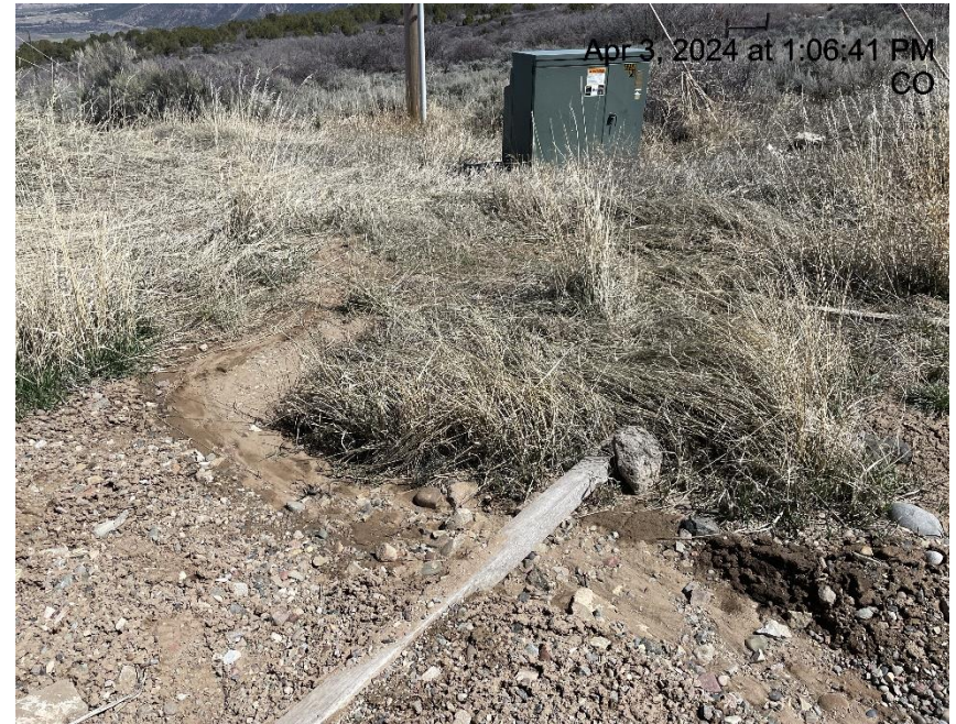
Photo # 2668 Erosion & transport of sediment off location into a vegetated area/sediment choking off vegetation /insufficient BMP's
