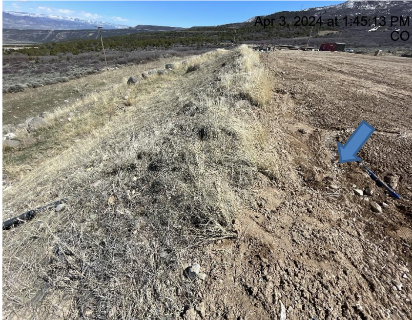
Photo # 2665 Drain/BMP needs maintenance/drain clogged with sediment (drain is near NW corner of location)
