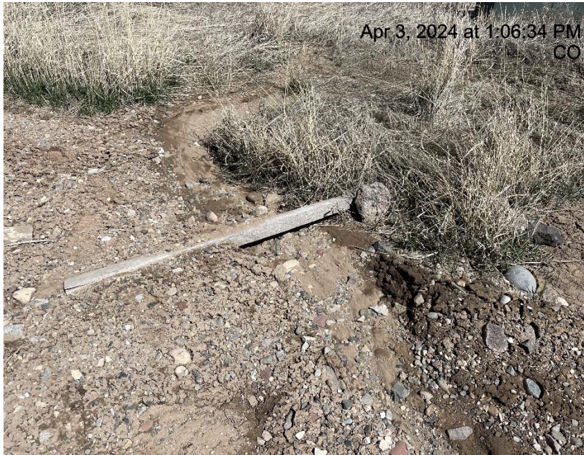
Photo # 2667 Erosion & transport of sediment off location into a vegetated area/sediment choking off vegetation /insufficient BMP's
