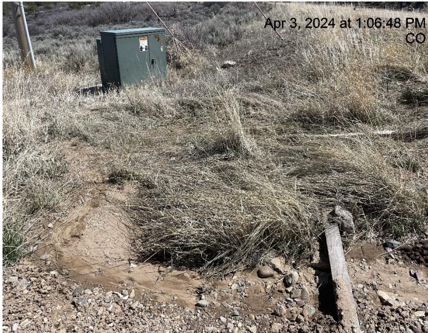
Photo # 2669 Erosion & transport of sediment off location into a vegetated area/sediment choking off vegetation /insufficient BMP's
