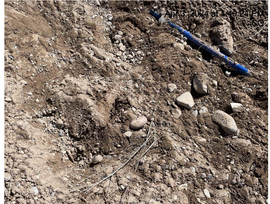
Photo # 2666 Drain/BMP needs maintenance/drain clogged with sediment (drain is near NW corner of location)
