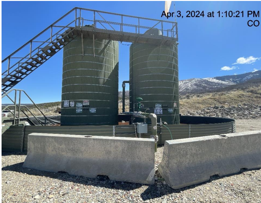
Photo # 2662 Tank battery lacks required signage
