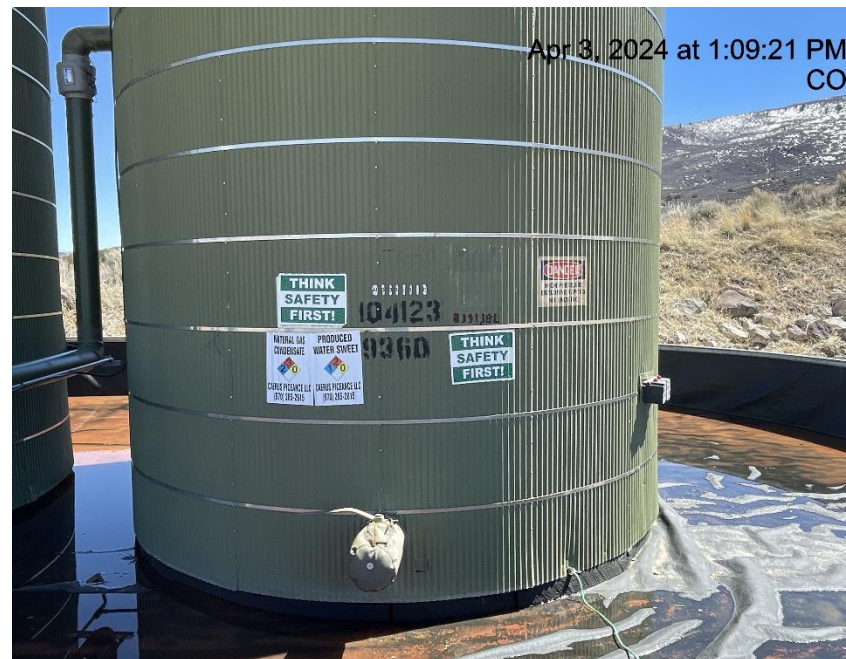
Photo # 2661 Production tank lacks some required info
