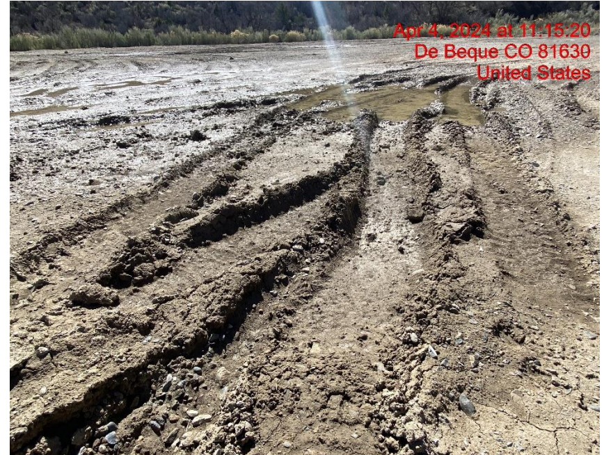
Lack of Stabilization – Photo #00380
