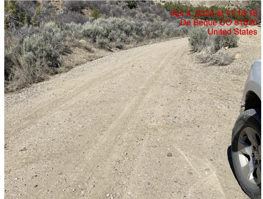
Insufficient Vehicle Tracking BMPs at Location Entrance/Exit – Photo #00388
