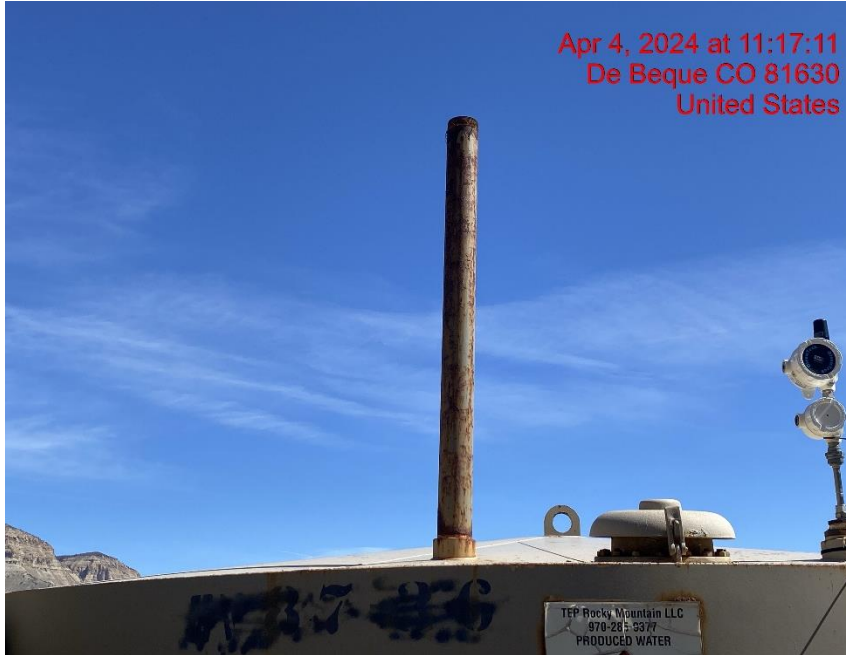
Open-Ended Vent/Wildlife Entry Hazard – Photo #00384
