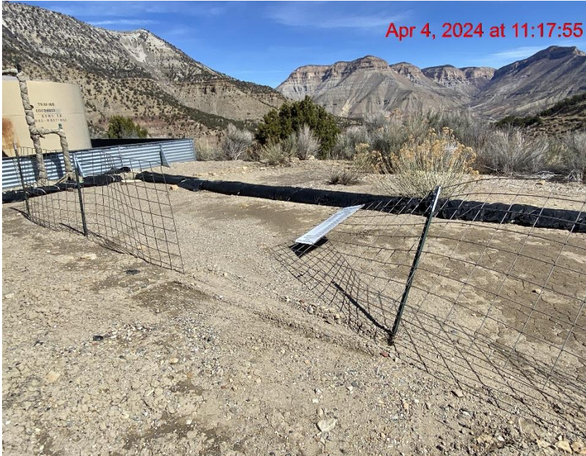
Damaged Fencing – Photo #00385
