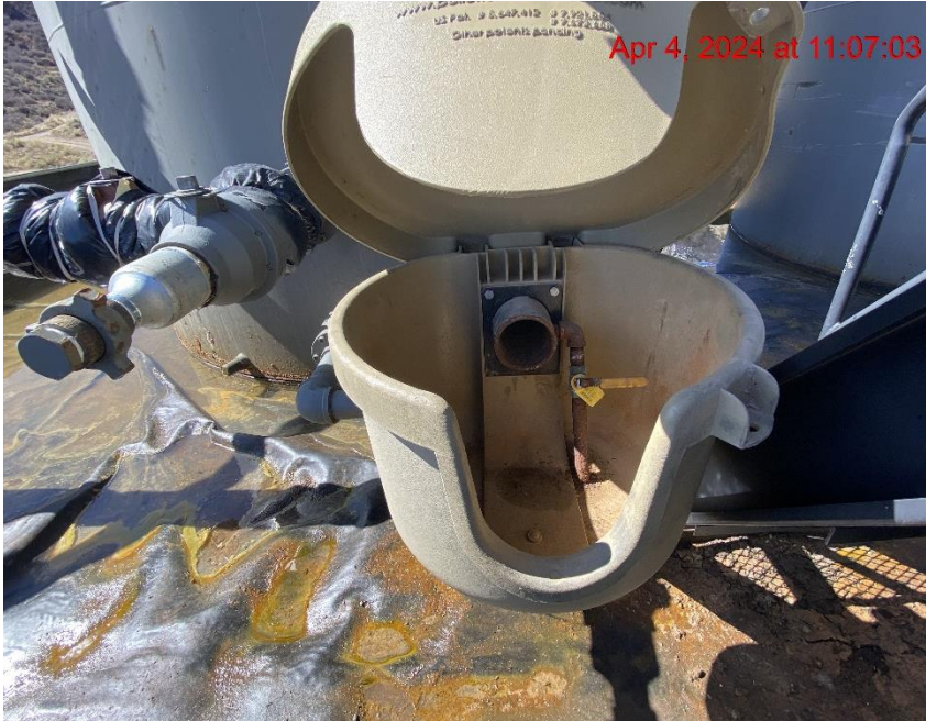
Open-Ended Load Line – Photo #00370
