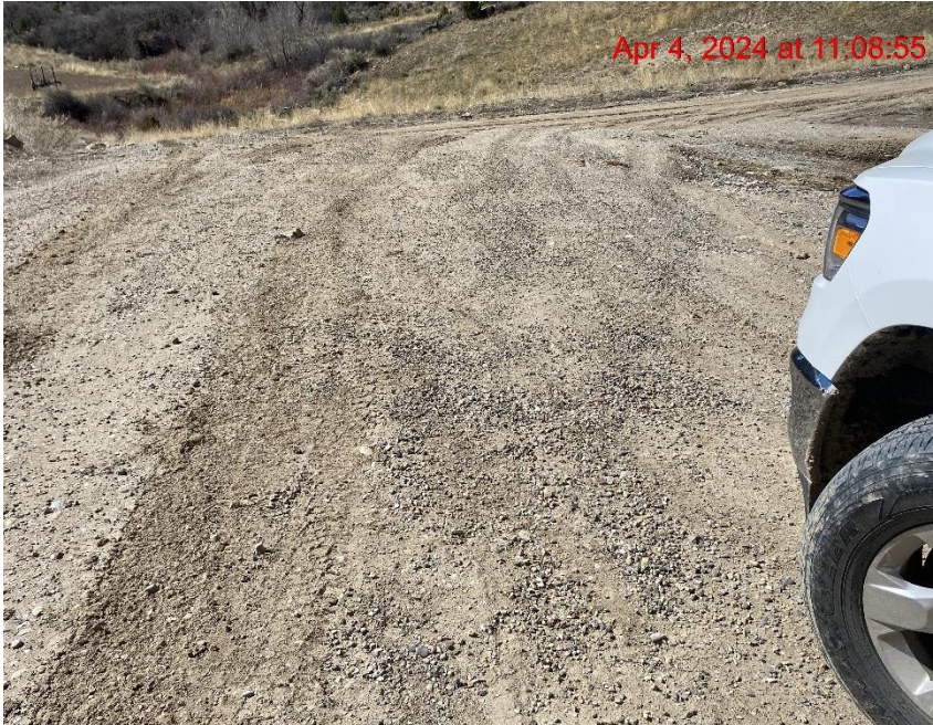
Insufficient Vehicle Tracking BMPs at Location Entrance/Exit – Photo #00377
