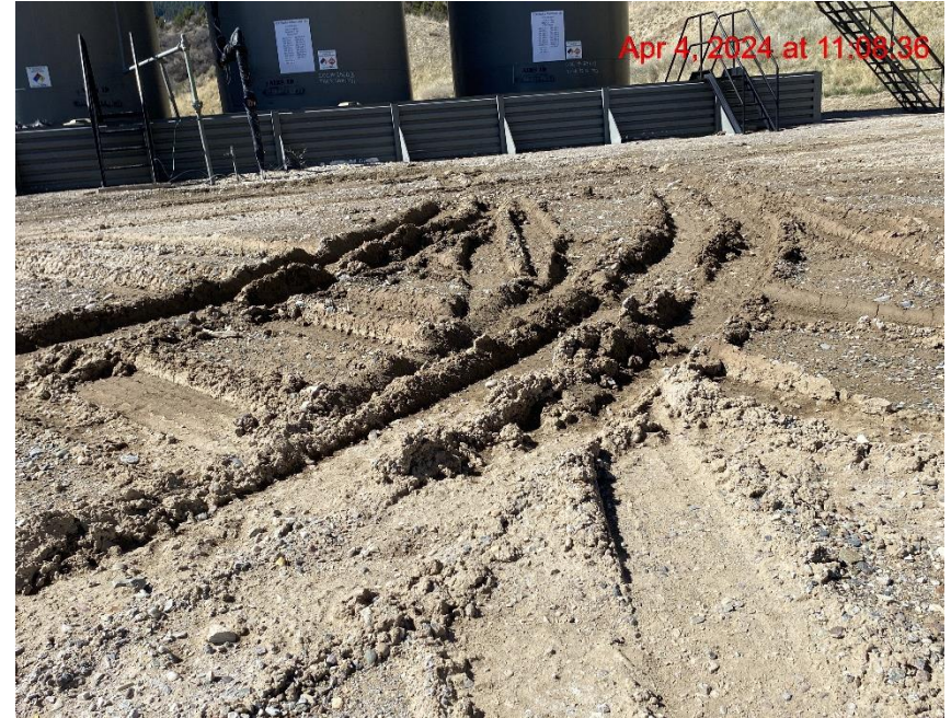
Lack of Stabilization – Photo #00376
