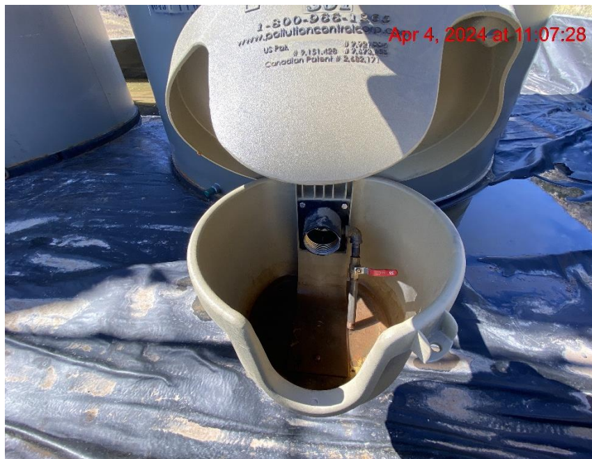
Open-Ended Load Line – Photo #00373
