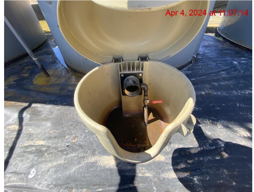
Open-Ended Load Line – Photo #00371
