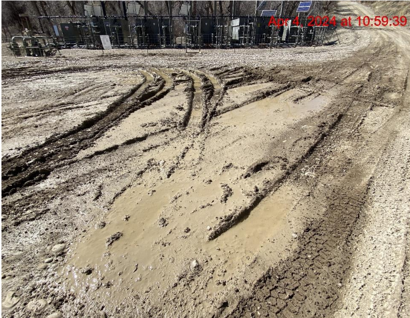
Lack of Stabilization – Photo #00361
