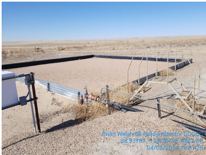
Old metal berms on south side of existing battery
