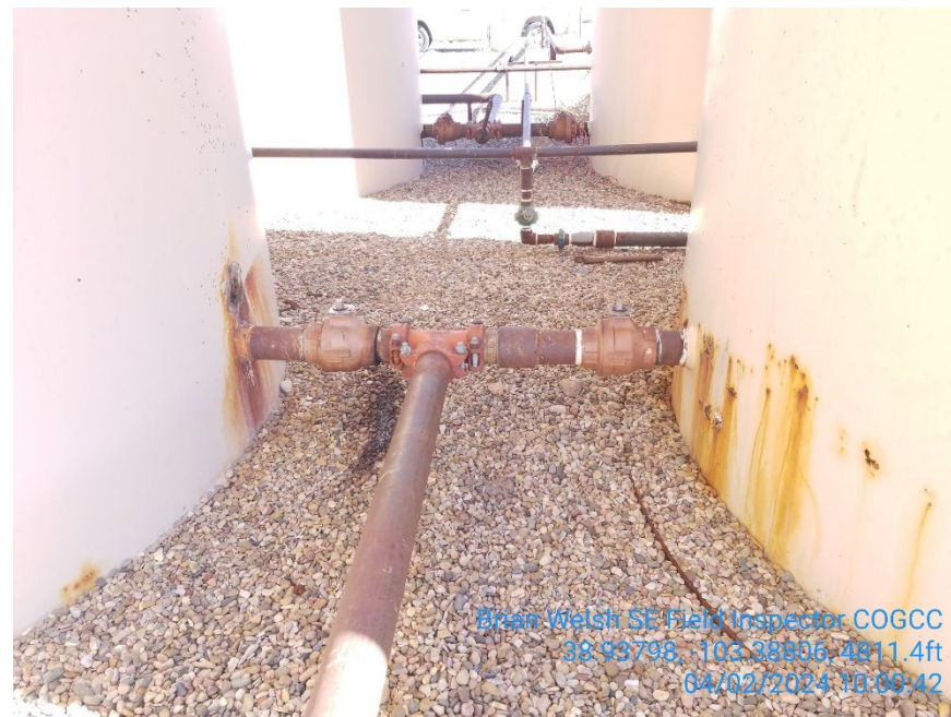
Picture showing how bad tanks are rotting
