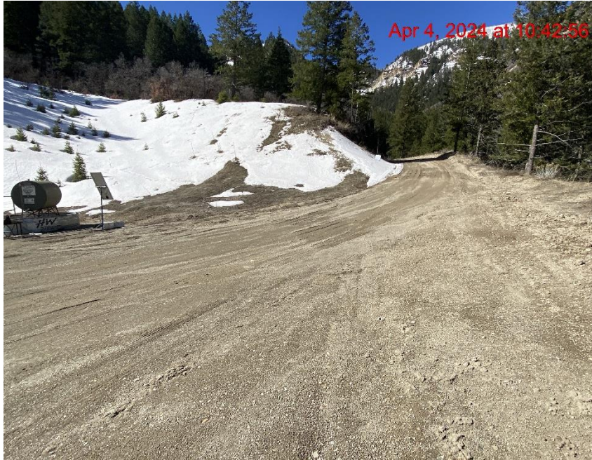
Insufficient Vehicle Tracking BMPs at Location Entrance/Exit – Photo #00356
