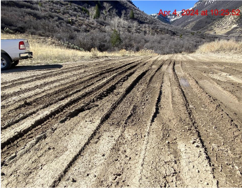
Lack of Stabilization/Insufficient Vehicle Tracking BMPs at Location Entrance/Exit – Photo #00342
