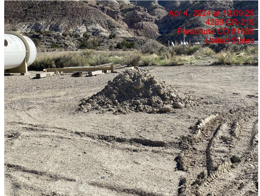
Unprotected Soil Stockpile Along Access Road– Photo #00336
