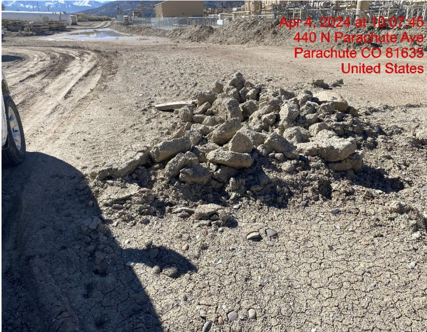
Unprotected Soil Stockpile – Photo #00334
