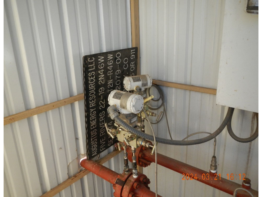
6. Digital gas meter inside meter shed.
