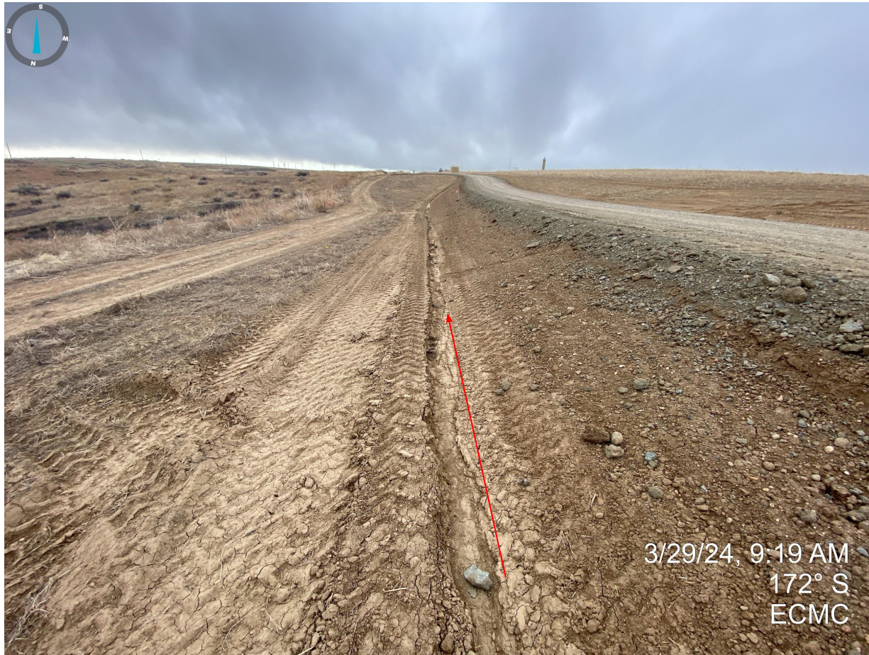
Photo 1. Erosion degradation (riling) occurring along the new access road.
