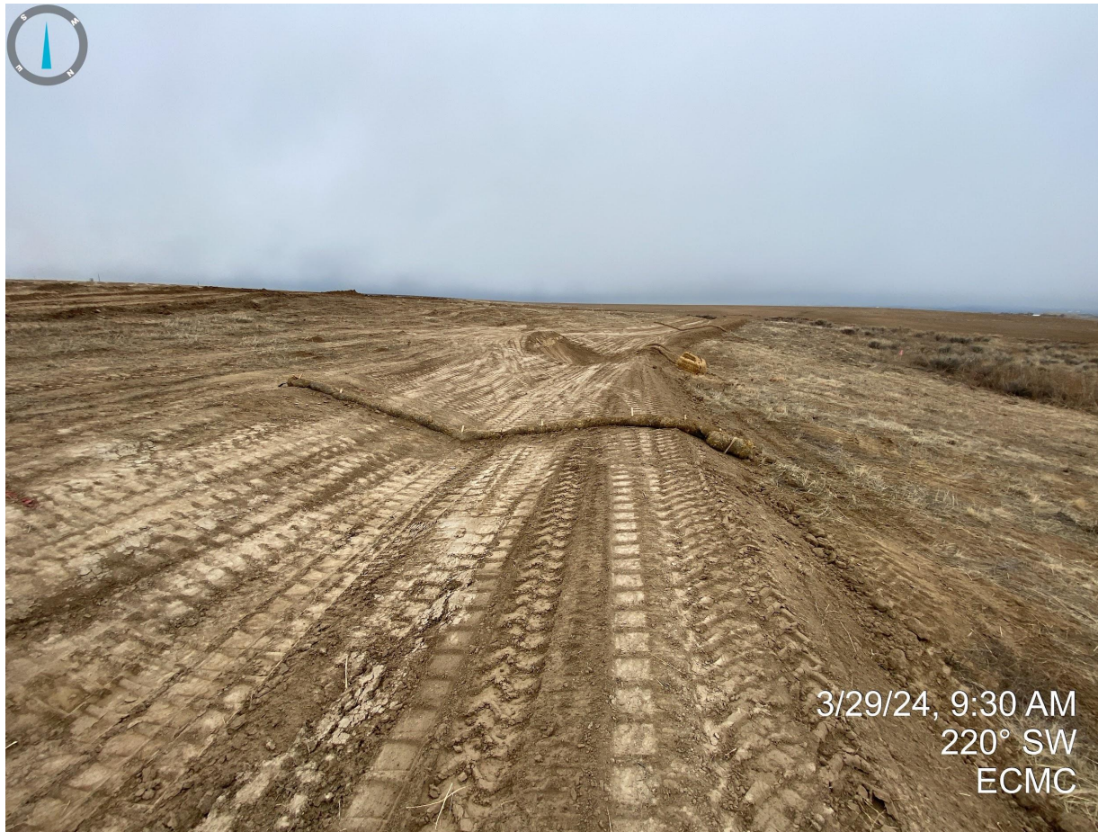
Photo 9. Taken along the northern perimeter of the construction area. A perimeter ditch and berm has been installed along the entire perimeter of the location with velocity checks (straw wattles) installed along gradients.
