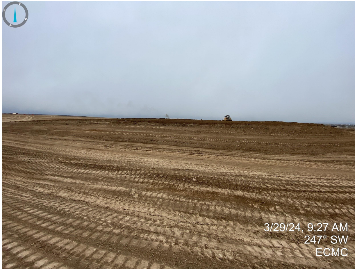
Photo 7. Taken near the northeast corner of the disturbance area. Photo illustrates the topsoil stockpile on the northern end of the location; crews were actively salvaging topsoil at the time of this inspection.
