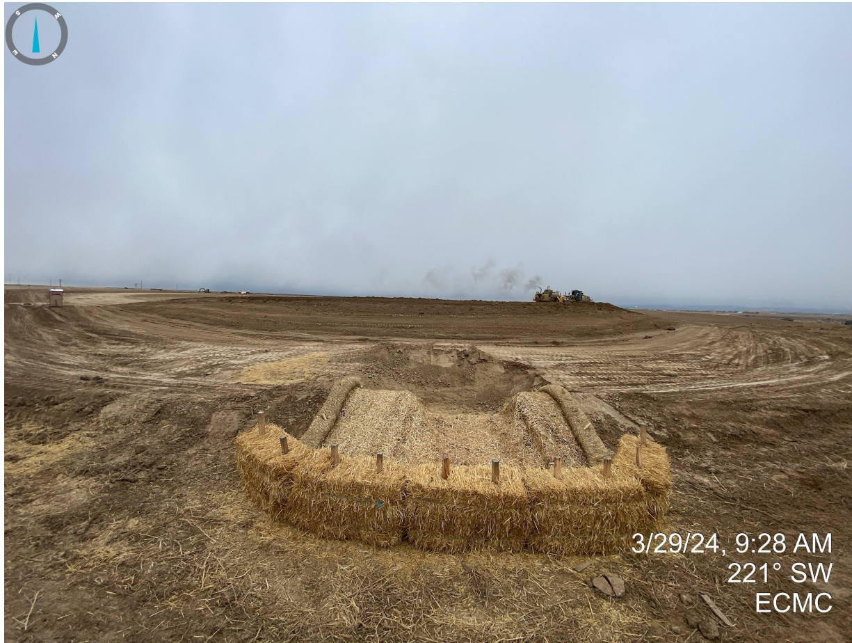
Photo 8. Taken near the northeast corner of the disturbance area. Photo illustrates a sediment trap with temporarily stabilized outlet protections.
