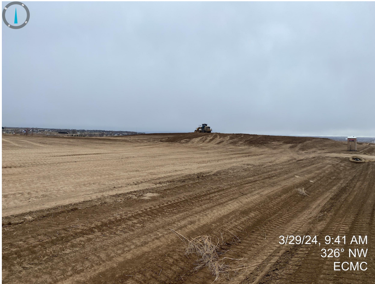
Photo 18. Taken near the location entrance. Photo illustrates overview of topsoil salvage operations and topsoil stockpile in the background. Operator shall ensure that all topsoil on location is salvaged in accordance with Rule 1002.b and that stockpiled soils are properly stabilized against wind and water erosion degradation.
