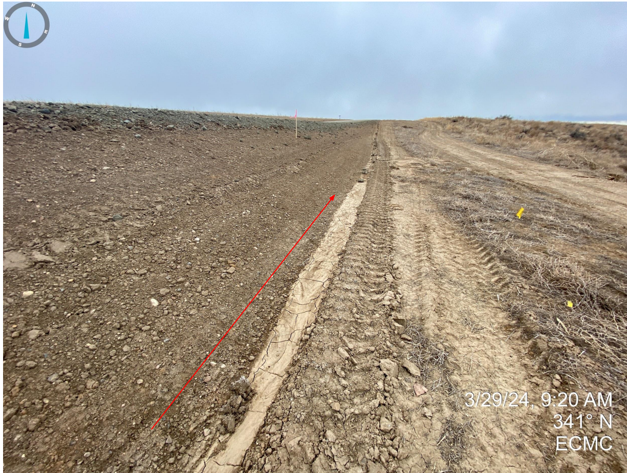
Photo 2. Erosion degradation (riling) and sediment deposition occurring along the new access road.
