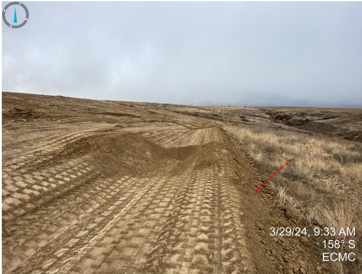
Photo 12. Taken near the western portion of the disturbance area. Some BMPs (sediment trap) remain in process. Portions of the perimeter berm do not appear to be properly stabilized as they have been left unconsolidated.
