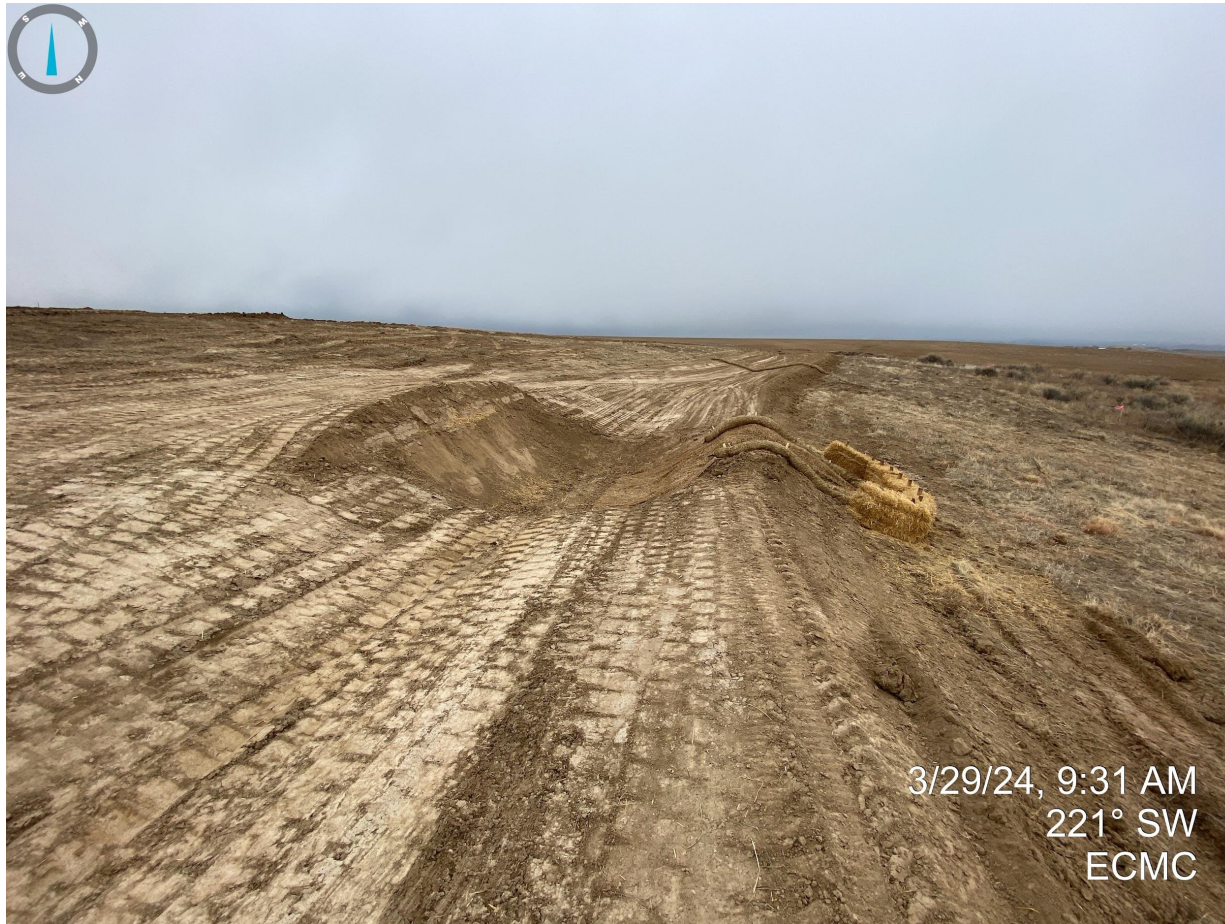
Photo 10. Taken near the northern portion of the disturbance area. Photo illustrates a sediment trap with temporarily stabilized outlet protections.
