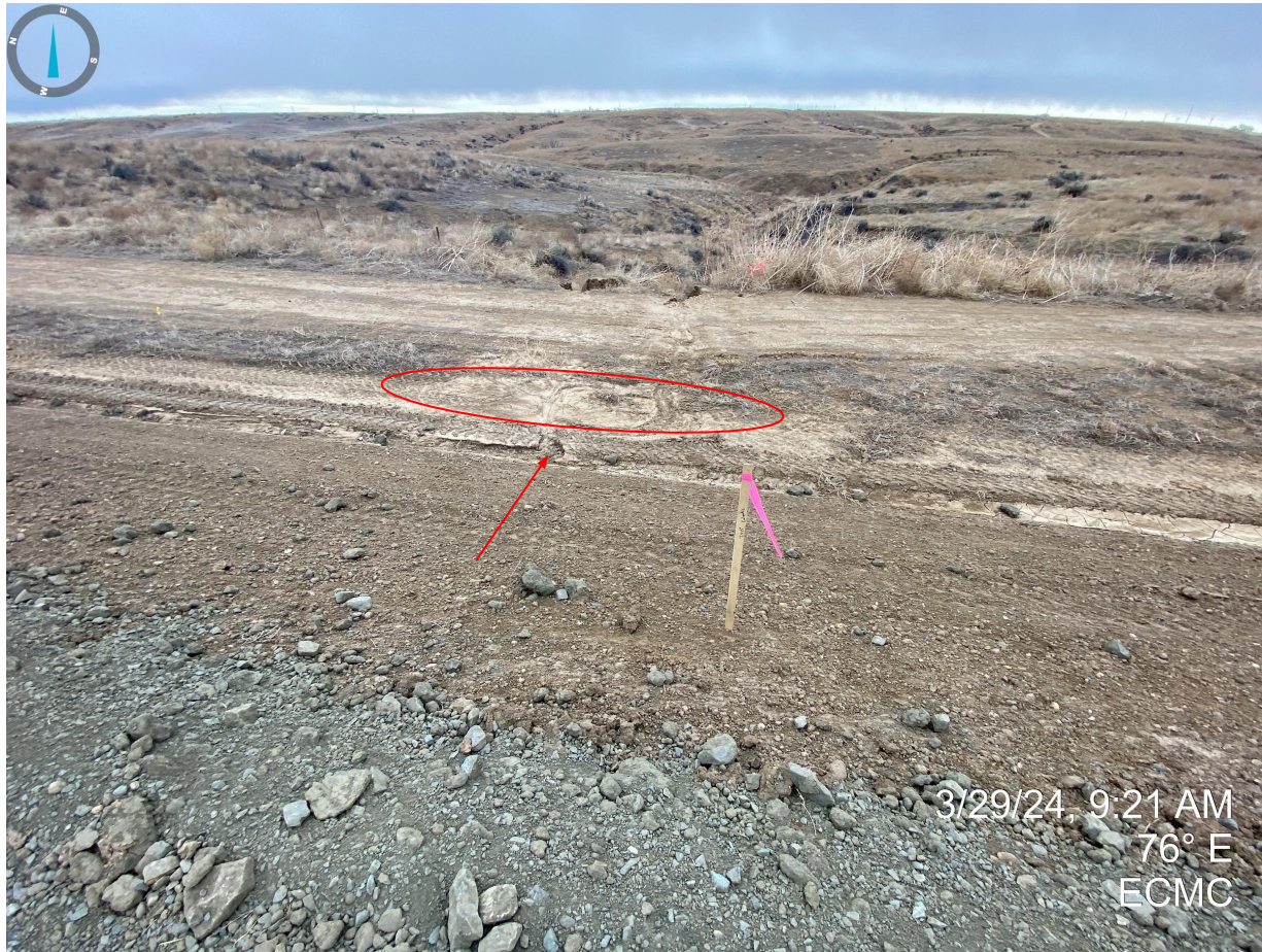
Photo 4. Sediment deposition observed on the east side of the new access road.
