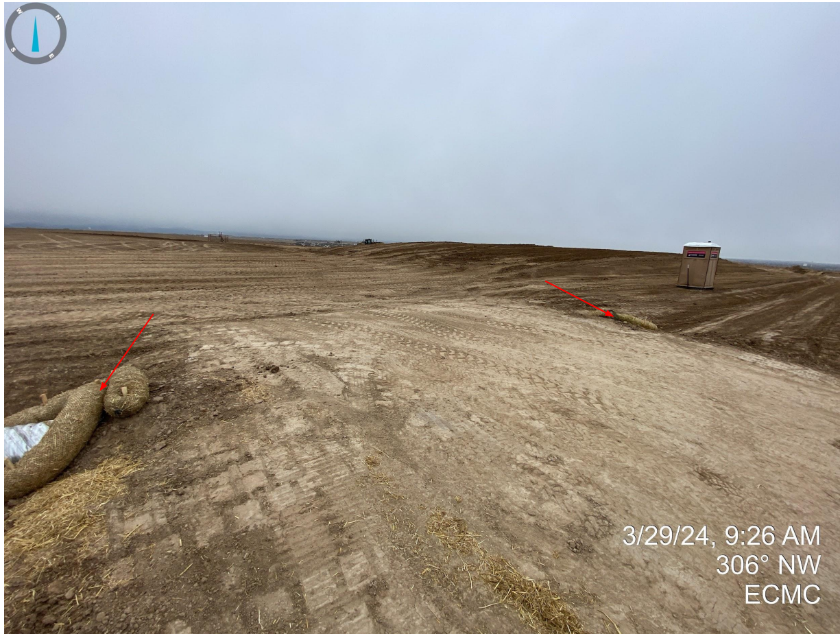
Photo 6. Temporarily stabilized inlets/outlets at culvert crossings observed at the location entrance.
