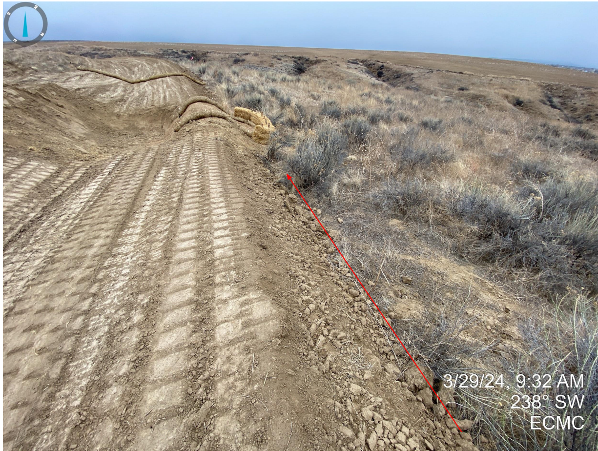
Photo 11. Taken near the northern portion of the disturbance area. Portions of the perimeter berm appear to be unconsolidated and require additional stabilization.
