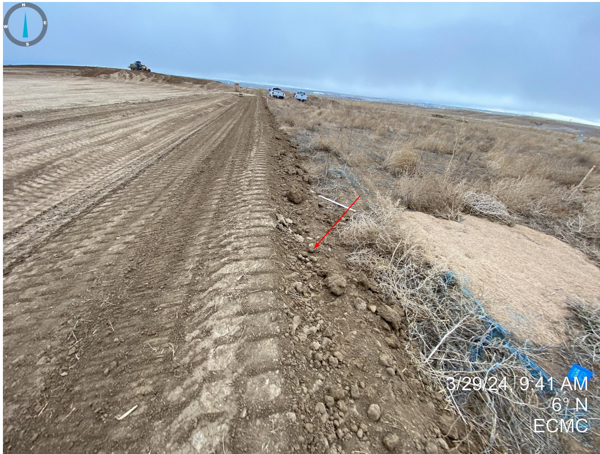
Photo 17. Taken from the eastern portion of the disturbance area. Photo illustrates that portions of the perimeter berm BMP do not appear to be properly stabilized as the soil has been left unconsolidated.
