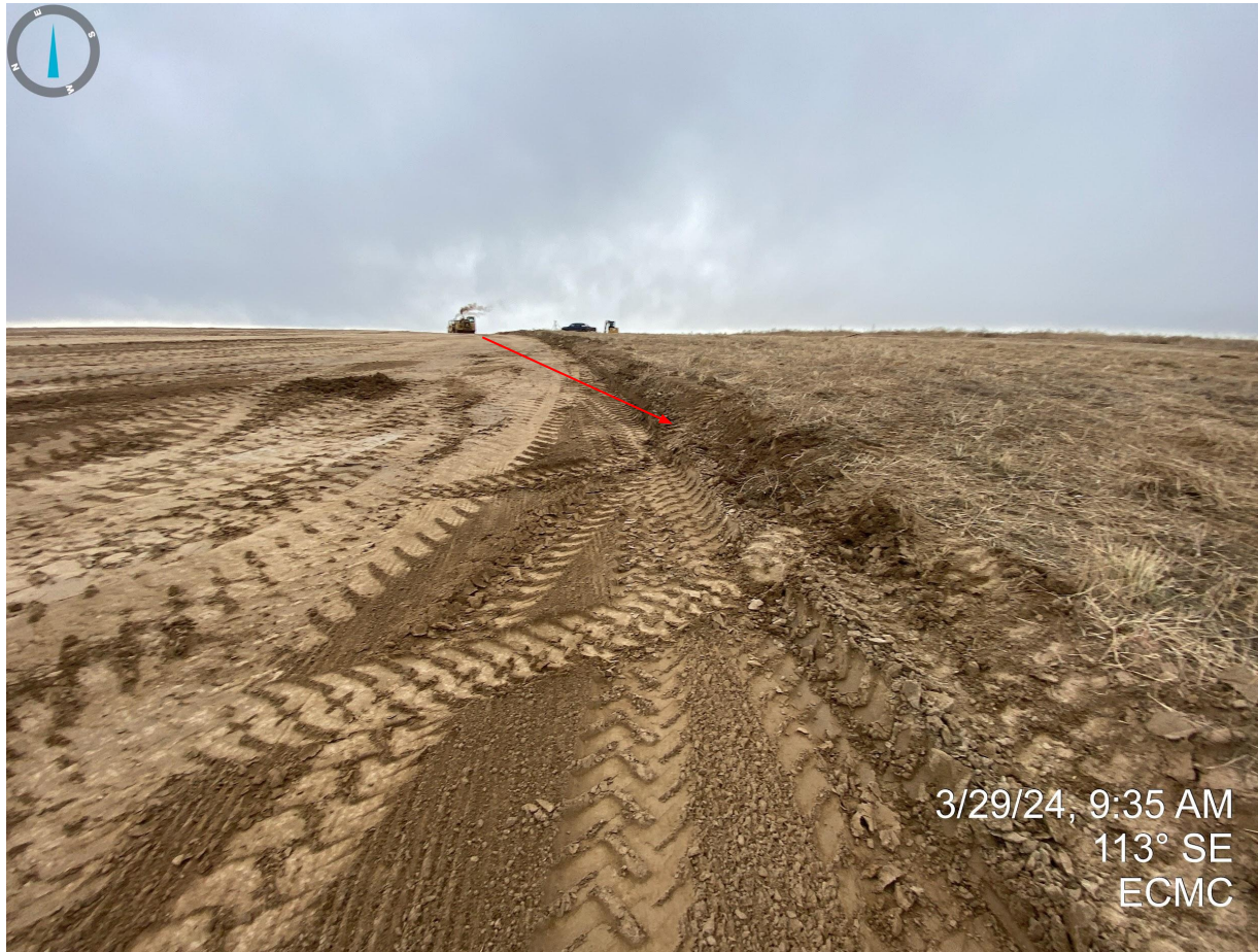
Photo 13. Taken near the southwest portion of the drilling pad construction. Photo illustrates topsoil salvage operations. Operator shall ensure that all topsoil on location is salvaged in accordance with Rule 1002.b.
