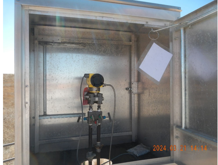
4. Digital gas meter inside meter box.
