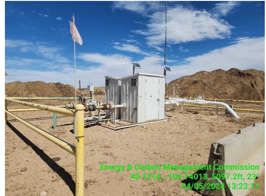
Photo 12 Gas Meter Run x 2 cards indicate current calibration.
