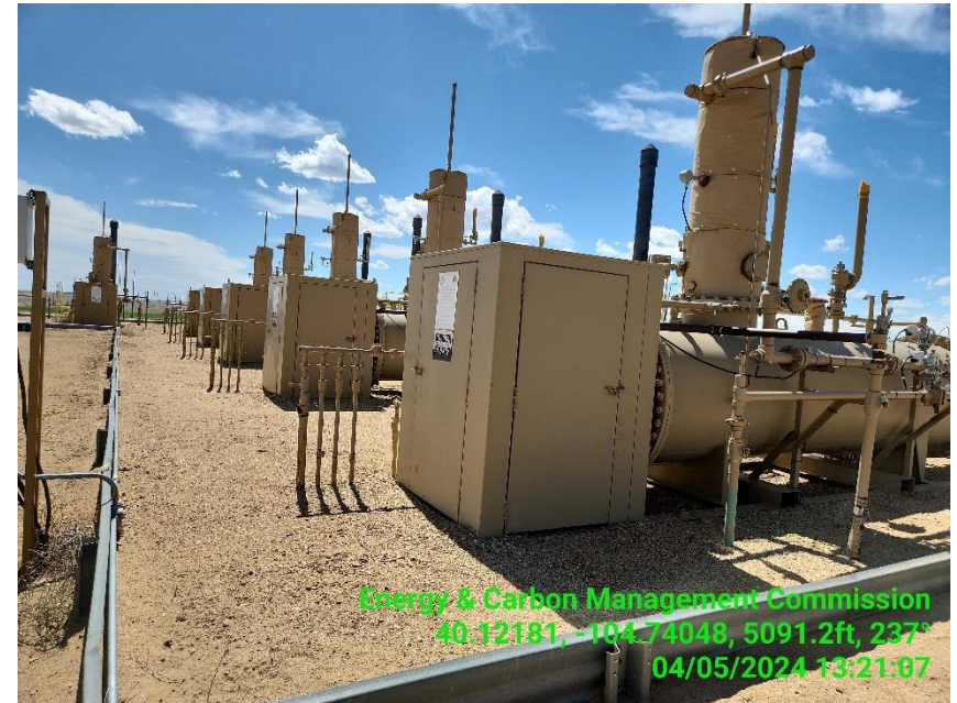
Photo 10 Horizontal Heated Separator.
