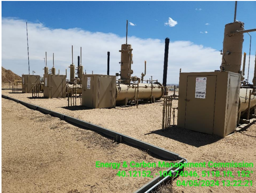
Photo 11 Horizontal Heated Separator.
