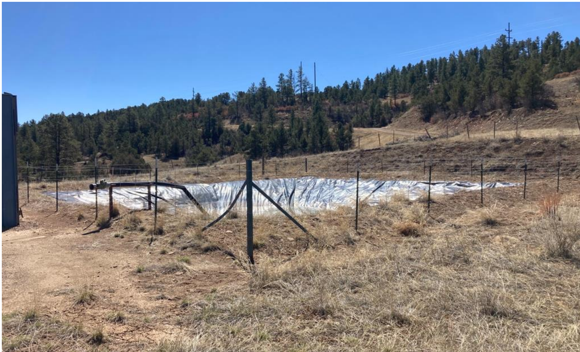
PHOTO 1: THE PIT FENCING HAS BEEN REPLACED WITH T-POSTS AND SMOOTH, BARBLESS WIRE.
