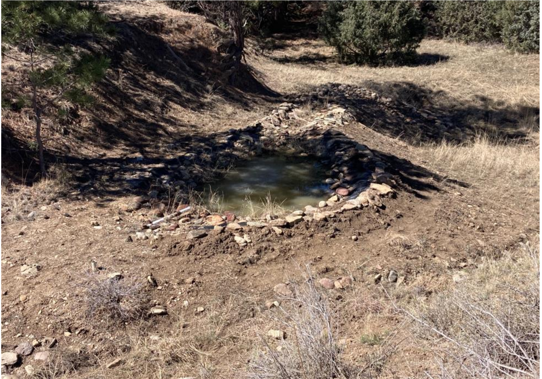
PHOTO 1: MAINTENANCE HAS BEEN PERFORMED TO THE DISCHARGE POINT. THE FENCING HAS BEEN REMOVED AND THE LINER RE-SET. ANY DISTIRBED GROUND HAS BEEN COMPACTED AND HAND SEEDDED TO PROMOTE STABILIZATION. OGRIS OPERATING IS PLANNING TO BEGIN OPERATIONS TO PERFORM MAINTENANCE/REPAIRS ON ALL DISCHARGE POINTS THIS SUMMER.
