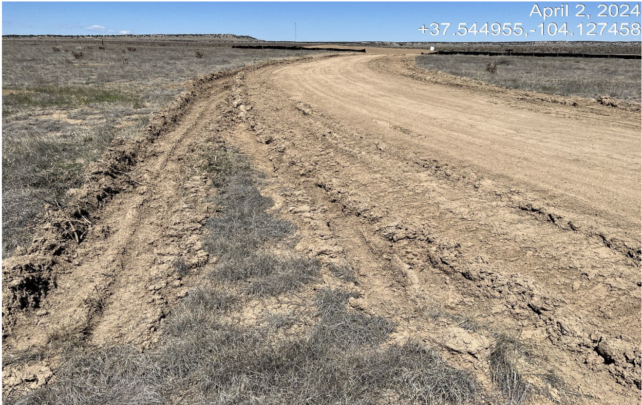
Photo 3. Facing northwest toward the access road. The side of the road needs to be seeded and stabilized and the road needs to be crowned and graveled. Previous corrective action was not completed.
