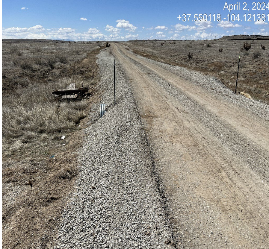
Photo 2. The drainage crossing has a large culvert but there is no outlet protection and loose gravel is falling into the culvert. Previous corrective action was not completed.
