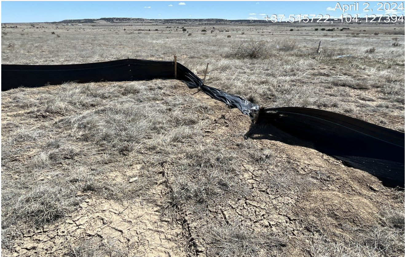
Photo 10 There are several area where the silt fence is not maintained. Previous corrective action was not completed.
