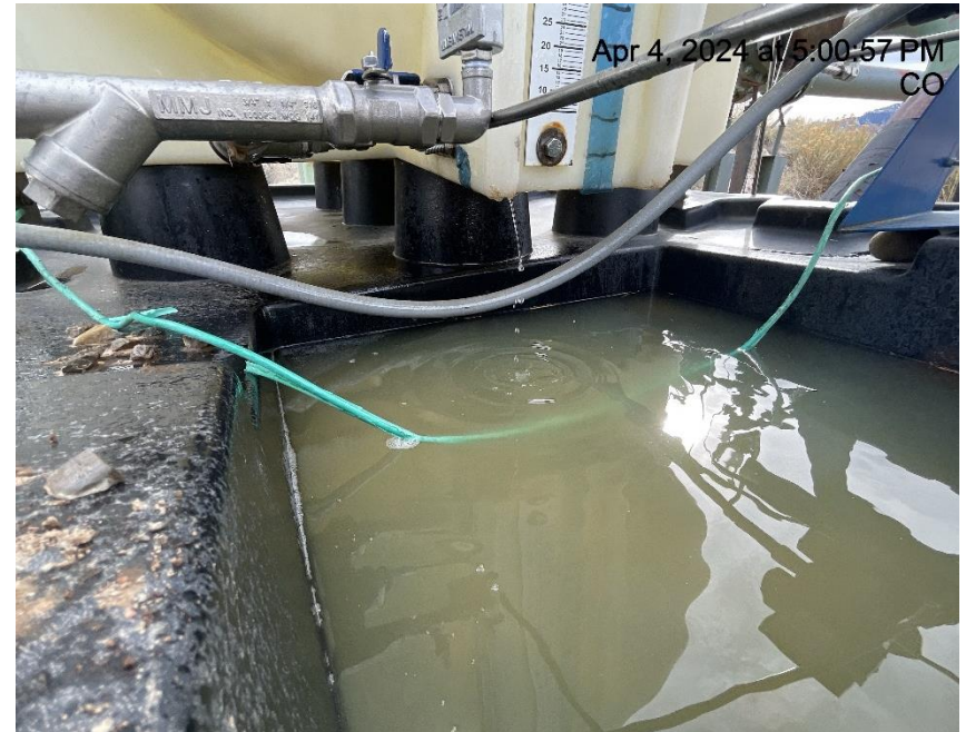
Photo # 2919 Mechanical condition – chemical tank leaking fluid
