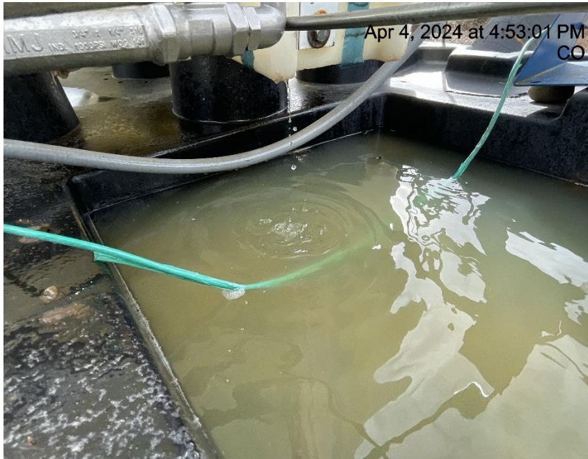
Photo # 2918 Mechanical condition – chemical tank leaking fluid
