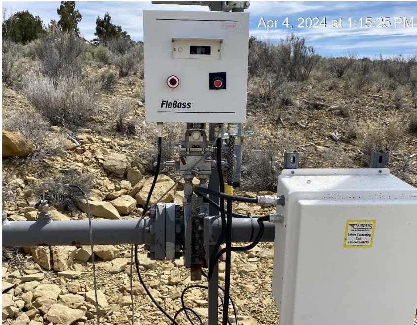
No visible display of gas meter calibration
