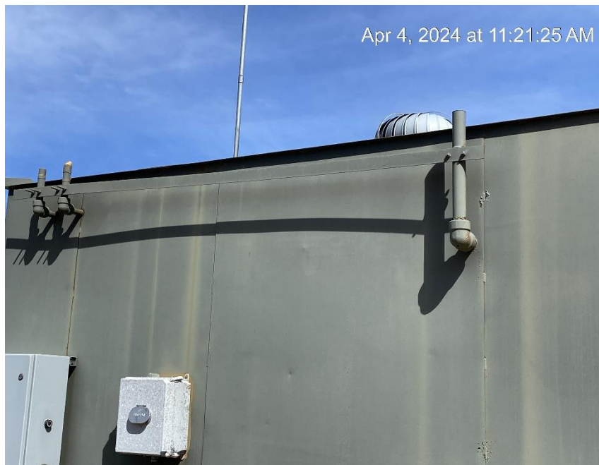
Relief risers missing rain protection
