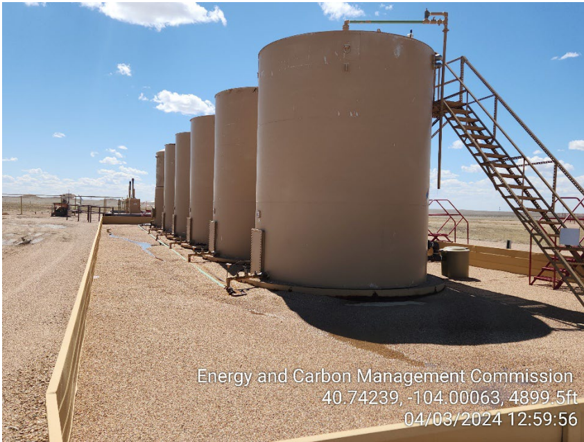
Photo 13 – Tank Battery
