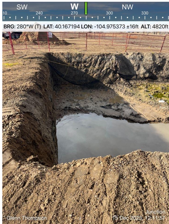
Ground Water in FL01 Excavation
