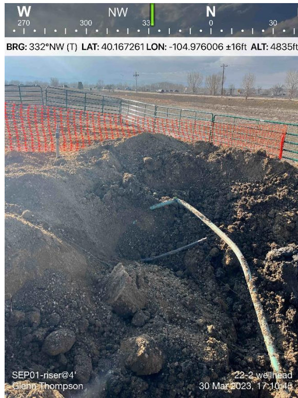
Separator Riser 01 Excavation
