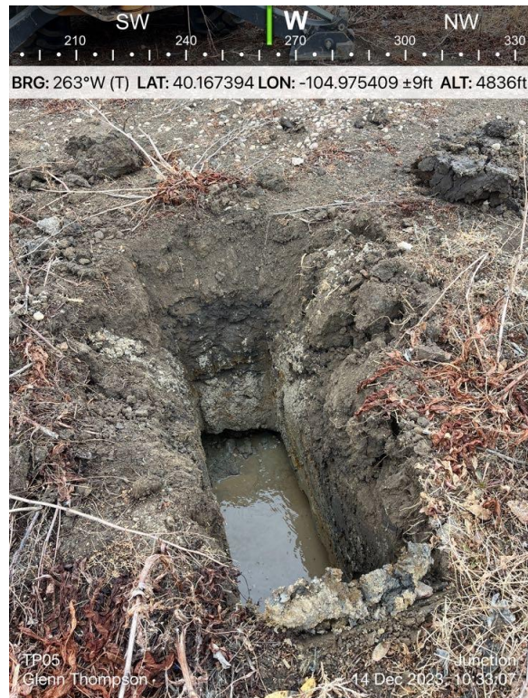
Ground Water in Test Pit 05 Excavation
