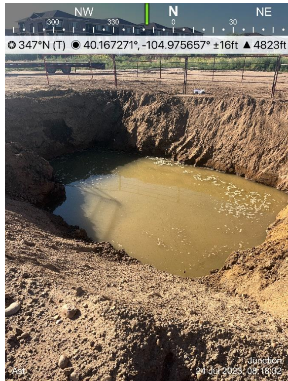
Groundwater in AST Excavation
