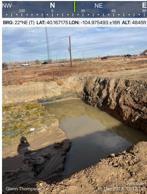
Ground Water in FL01 Excavation
