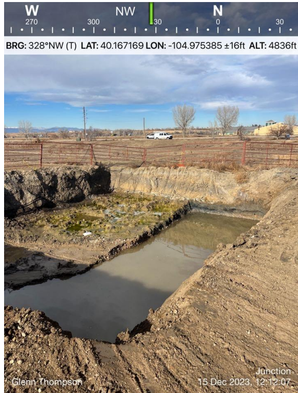
Ground Water in FL01 Excavation
