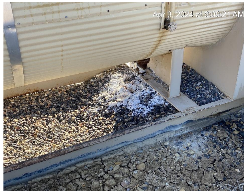
Separator leak and impacted soil
