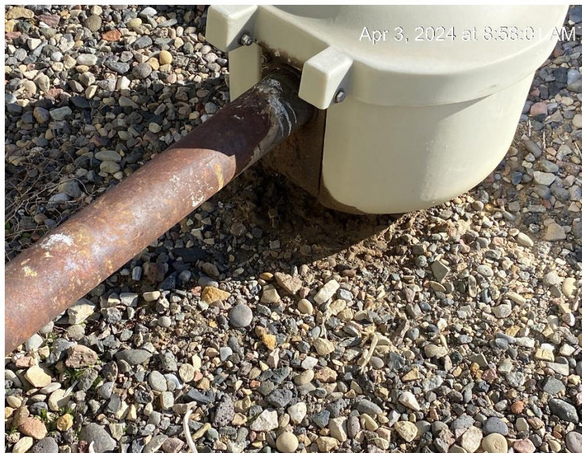
Oily waste under load pot
