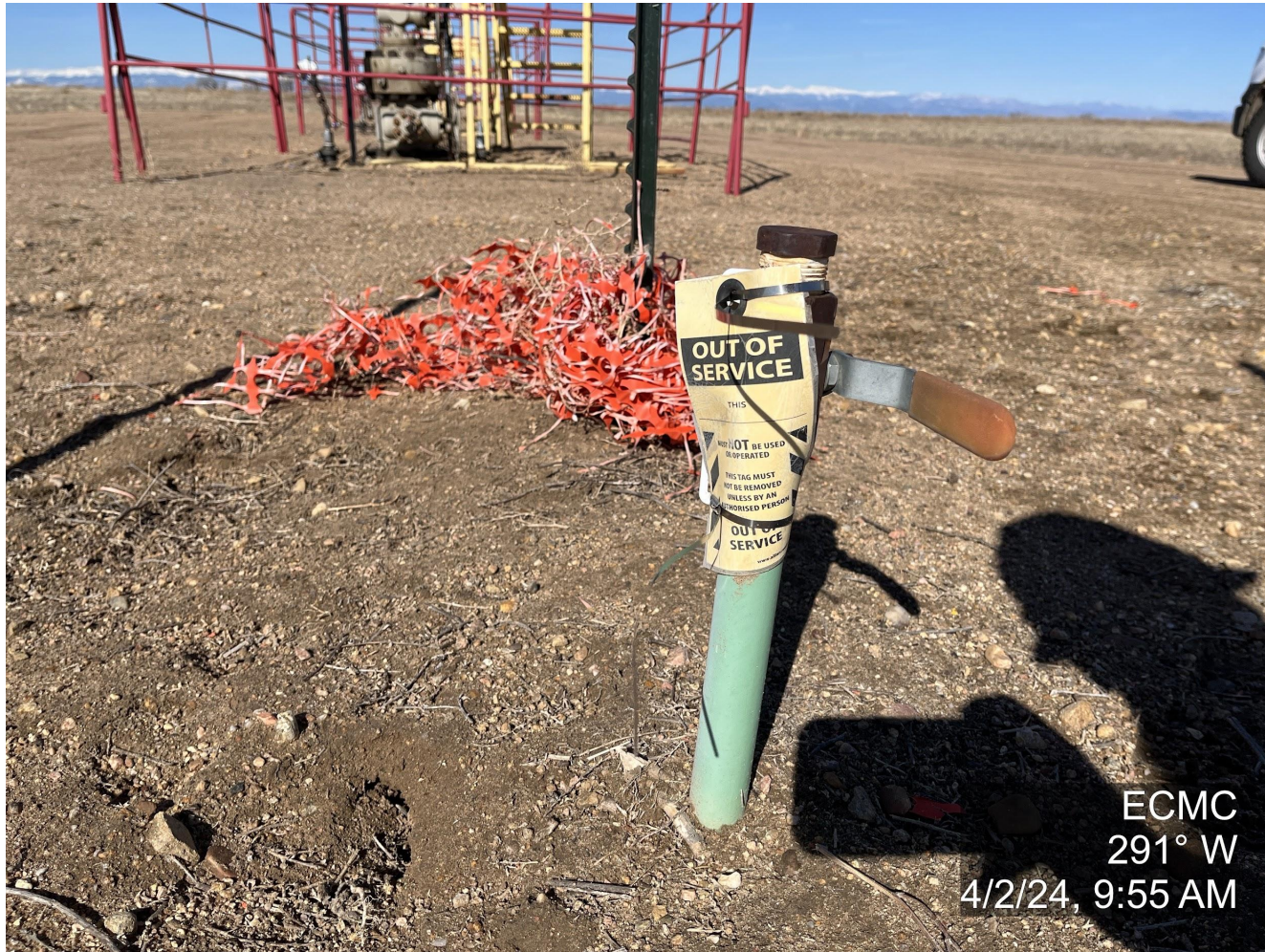
Photo 1. The photo was taken at the well location facing West. The photo illustrates the remaining rise at the plugged and abandoned well.
