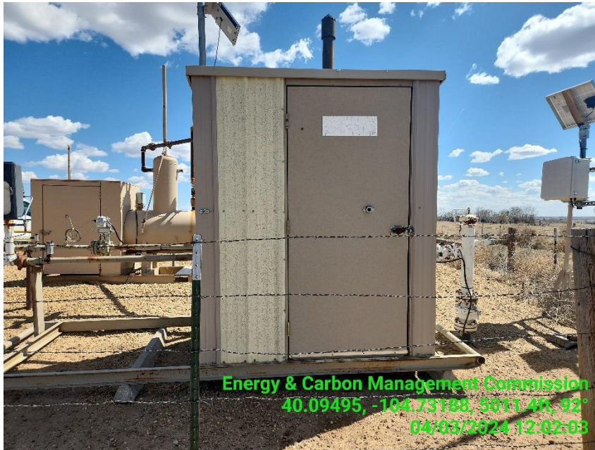
Photo 5 Gas meter Run is SI/LOTO.
