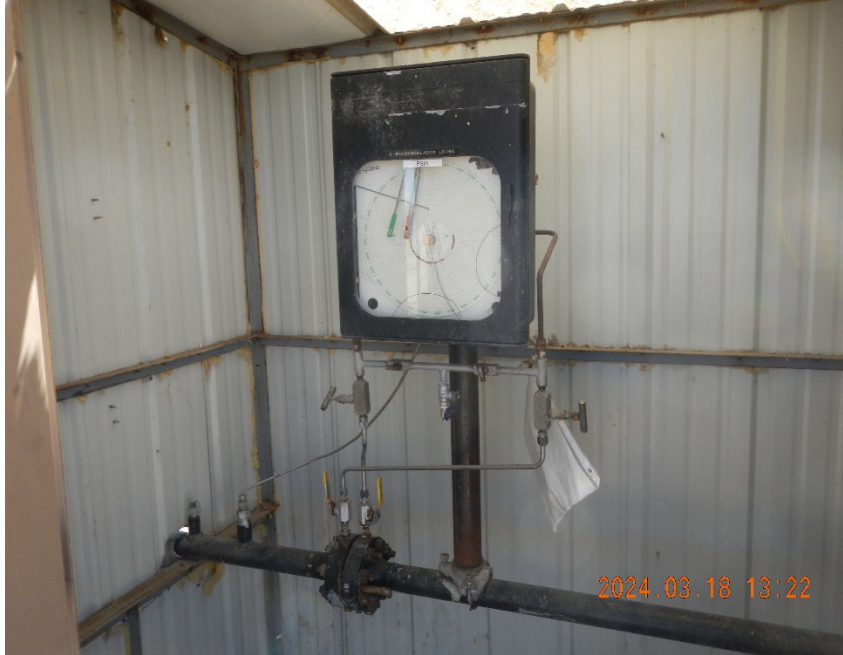
5. Gas meter inside remote shared meter shed.
