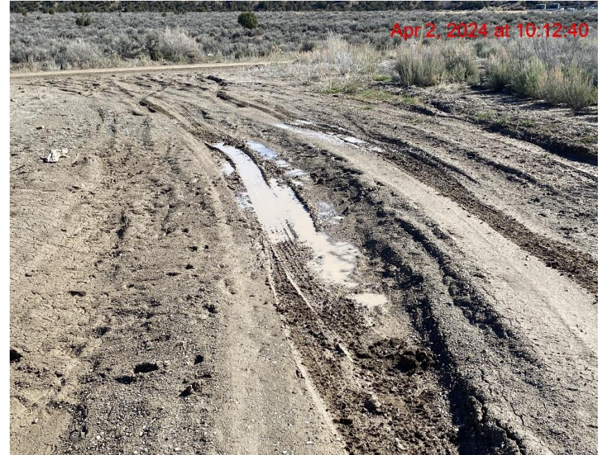
Lack of Stabilization/Insufficient Vehicle Tracking BMPs at Location Entrance/Exit – Photo #00286
