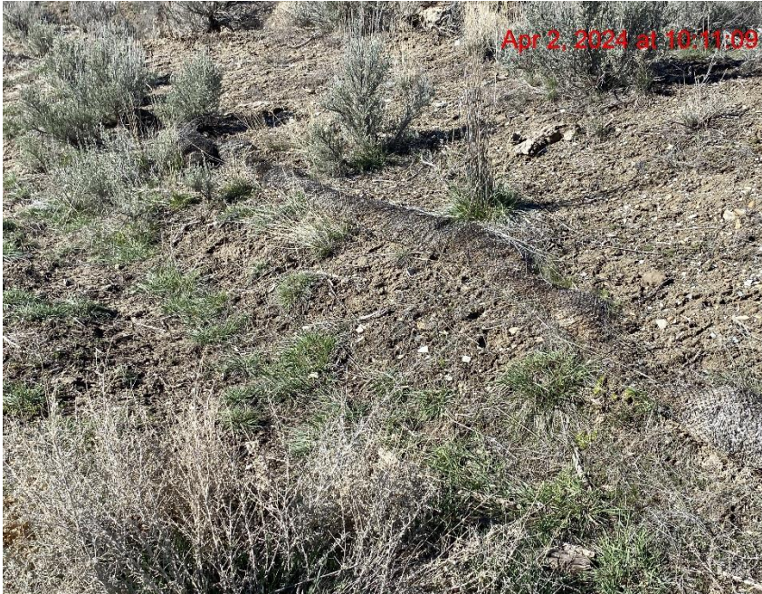
Degraded Waddles on Perimeter of Location – Photo #00285
