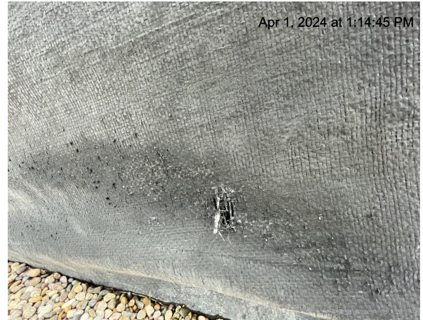
Photo # 2240 Hole in liner/liner needs maintenance & liner showing signs of deterioration
