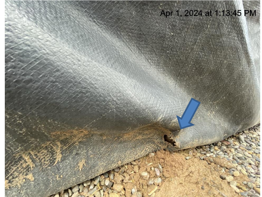
Photo # 2244 Hole in liner/liner needs maintenance
