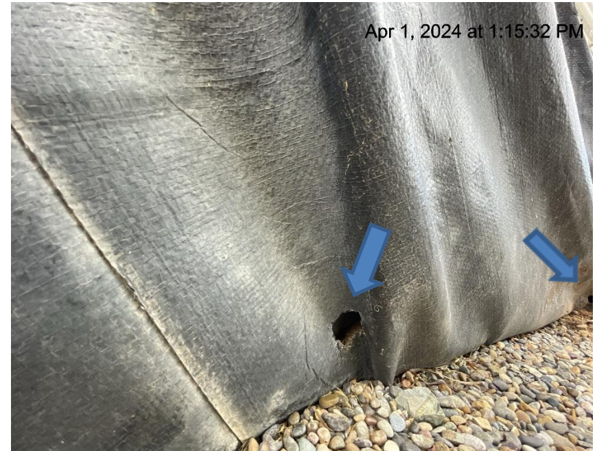
Photo # 2242 Holes in liner/liner needs maintenance
