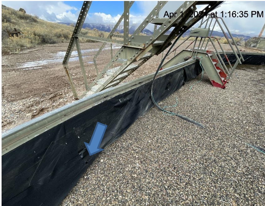
Photo # 2245 Hole in liner/liner needs maintenance
