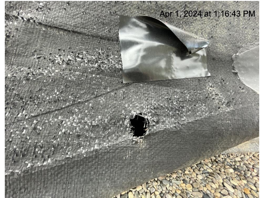
Photo # 2246 Hole in liner/liner needs maintenance & liner showing signs of deterioration
