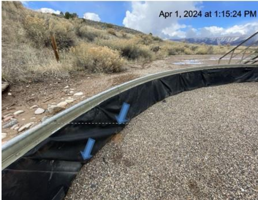
Photo # 2243 Holes in liner/liner needs maintenance
