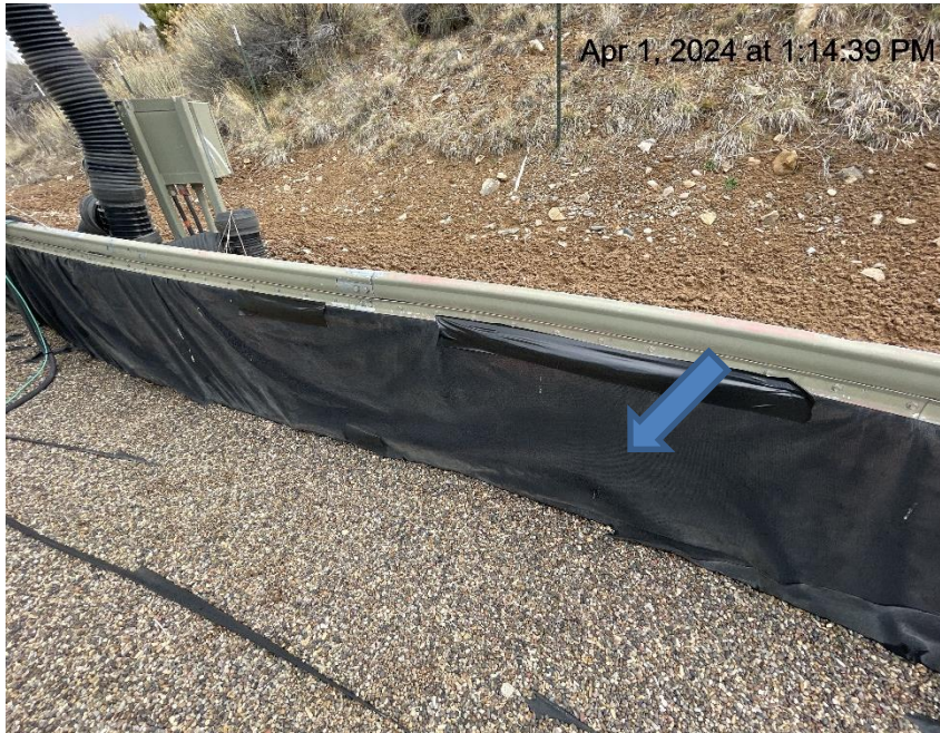
Photo # 2239 Hole in liner/liner needs maintenance
