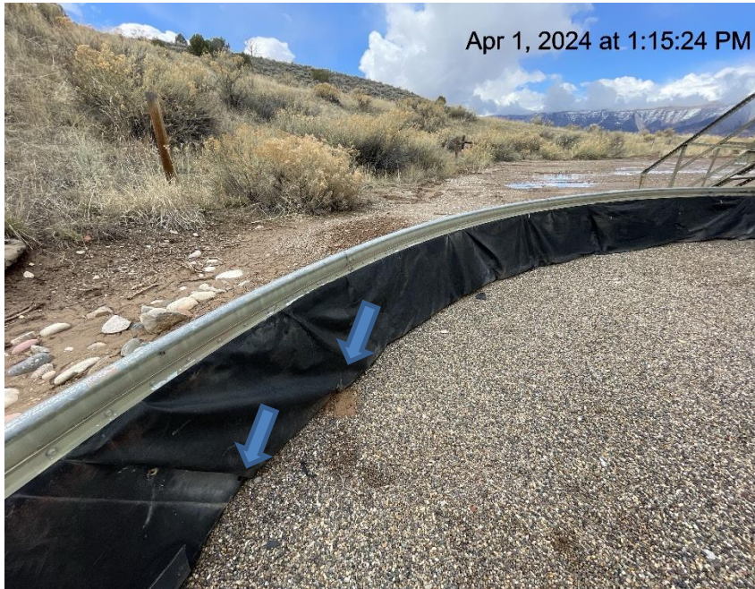
Photo # 2241 Holes in liner/liner needs maintenance
