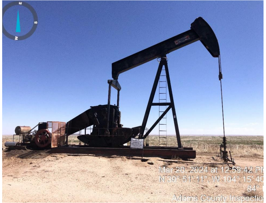
Photo #6 Pump jack.
