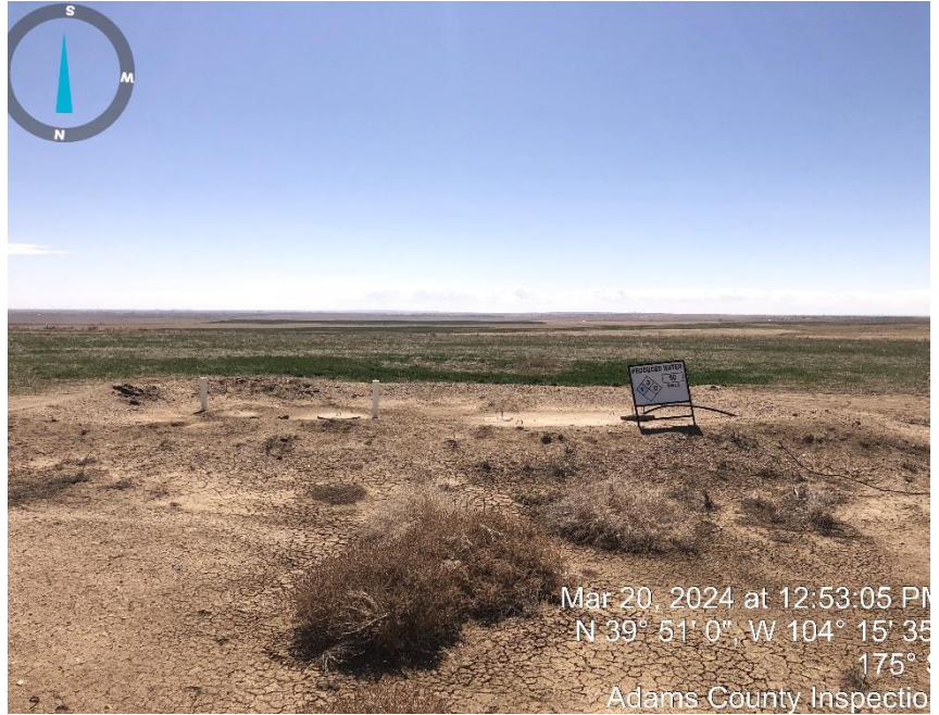
Photo #4 P/W Vault.
