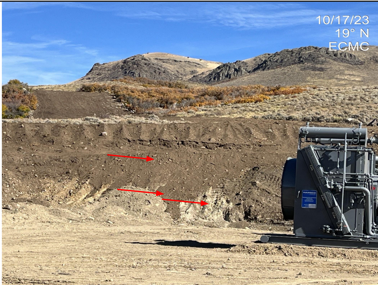
Photo 8: Photo taken from the north end of the Location, facing northeast. Photo shows cut slopes of the Location lack stabilization. BMPs to minimize erosion, degradation and sediment transport are missing or insufficient; BMPs to manage runoff/runoff along eastern perimeter missing or insufficient. Photo also shows the mixing of soil horizons, such as the topsoil; Operator failed to salvage all topsoil on the Location; Operator failed to separate and store soil horizons separately based on changes in physical characteristics (such as organic content, color, texture, density or consistency).
