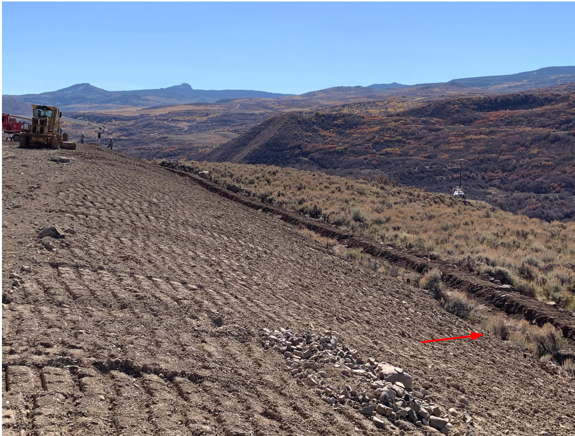
Photo 9: Photo taken from the southwest end of the Location, facing southeast. Photo example showing surface roughening (tracking) implemented on fill slopes. Photo also example showing ditch/berm constructed along the perimeter of the Location; BMPs had been constructed with use of topsoil material. Photo also shows intact vegetation (arrow, shrubs) along the perimeter of the Location, partially covered with fill material, indicating that not all topsoil had been salvaged and segregated during construction.
