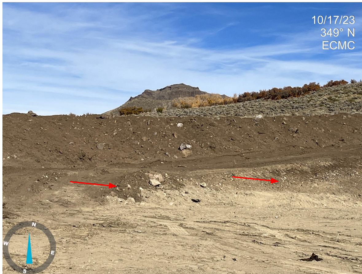
Photo 11: Photo taken from the north end of the Location, facing northwest. Photo shows the topsoil stockpile. Stockpile bare, unstabilized and at risk from wind and water erosion; BMPs to minimize erosion and degradation missing from the stockpile; control measures to manage stormwater runoff and minimize sediment transport are also missing along the perimeter of the stockpile. Photo also shows the mixing of different soil horizons, such as the topsoil; Operator failed to salvage all topsoil on the Location; Operator failed to separate and store soil horizons separately based on changes in physical characteristics (such as organic content, color, texture, density or consistency).
