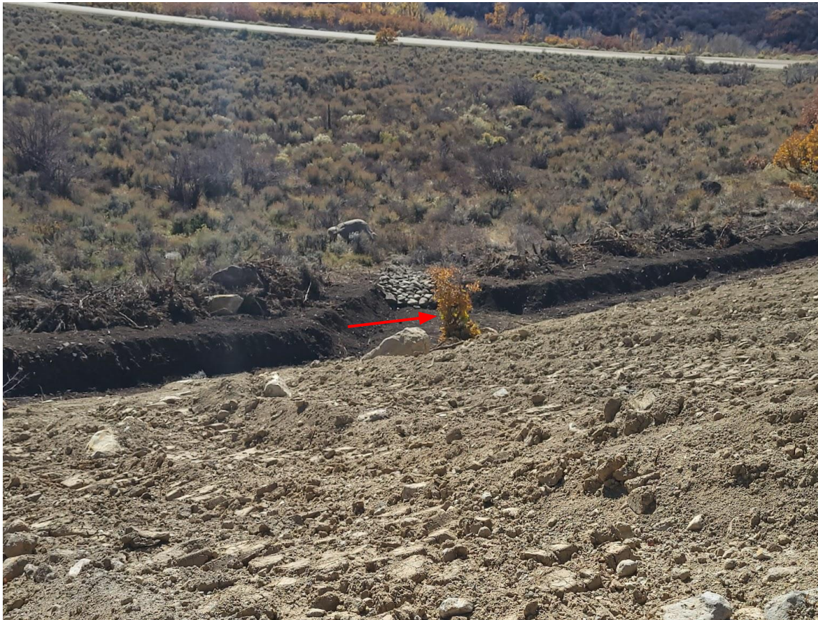
Photo 10: Photo taken from the southeast end of the Location, facing southeast. Photo shows 1 of the 2 sediment traps on the Location, as well as the ditch/berm along the perimeter; BMPs had been constructed with use of topsoil material. Photo also shows intact vegetation (arrow, tree) along the perimeter of the Location, partially covered with fill material, indicating that not all topsoil had been salvaged and segregated during construction.
